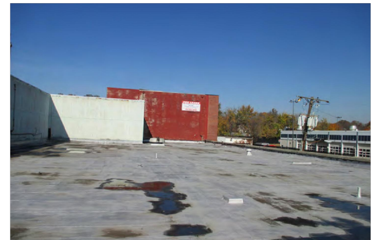
7 ROOF NORTH VIEW
