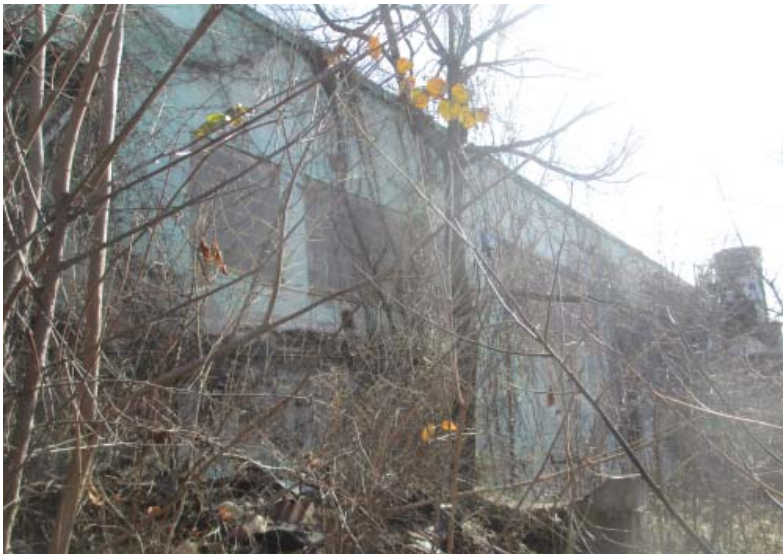
2. VIEW OF WEST (REAR) FACADE FROM NORTH OF SITE
