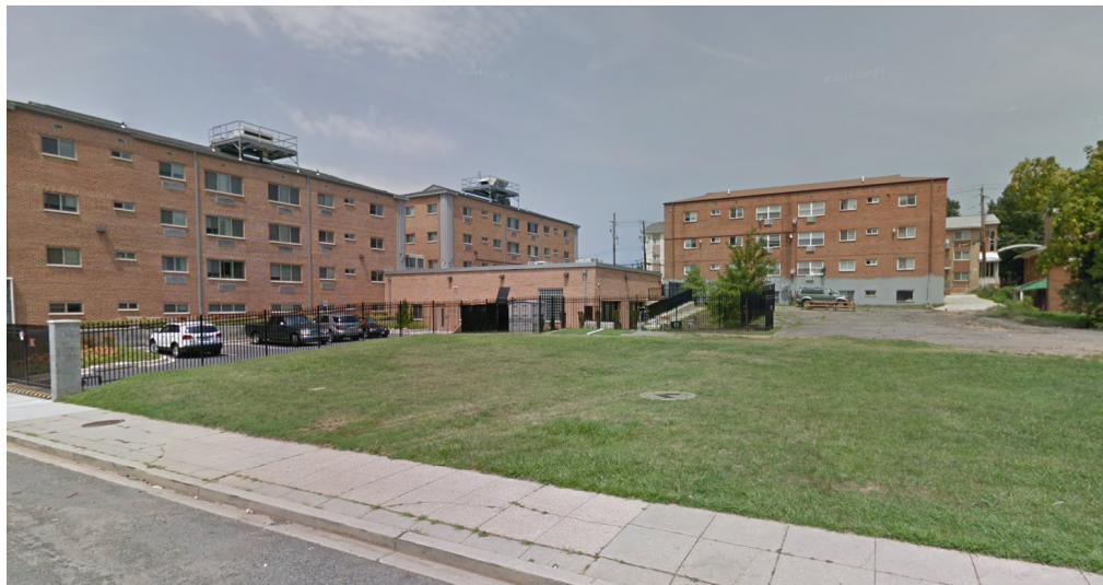
5. Site, Looking Northwest
