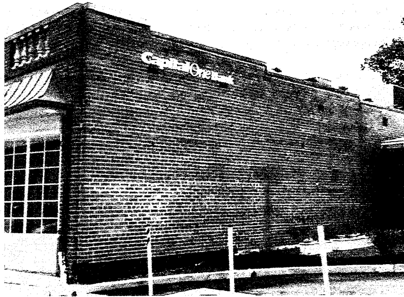
North side wall of 4860 Massachusetts Avenue, NW
