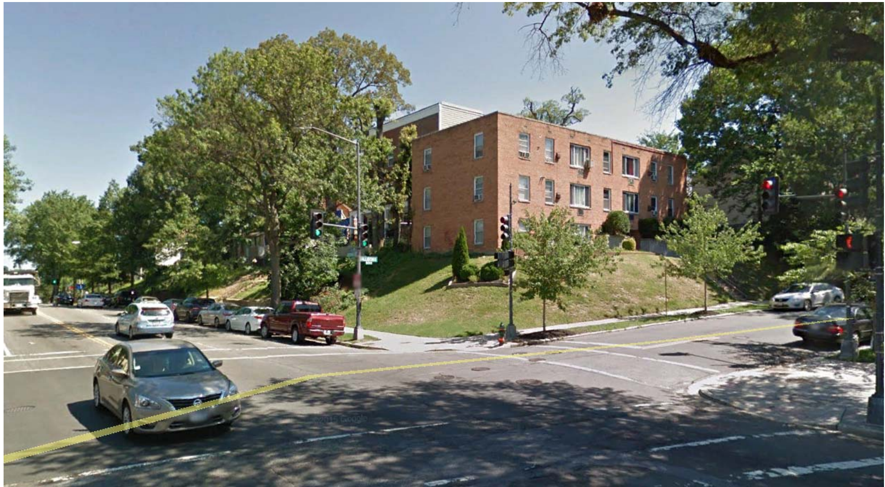
Multifamily east side of Georgia Avenue- North on Allison Street
