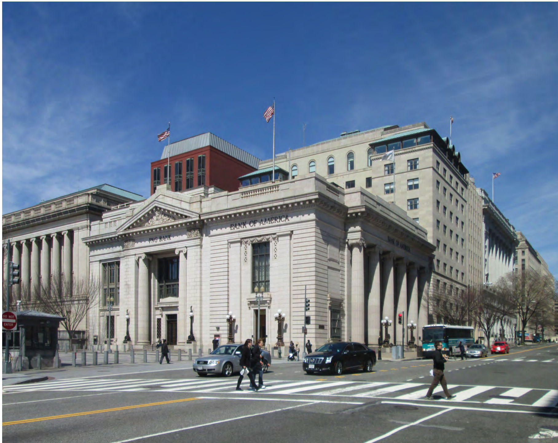
C. Pennsylvania Ave. and New York Ave. Looking Northwest
