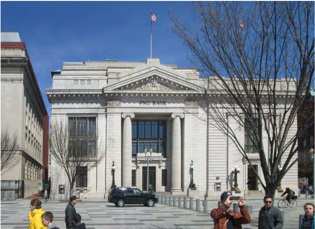
B. From Treasury Building Looking North
