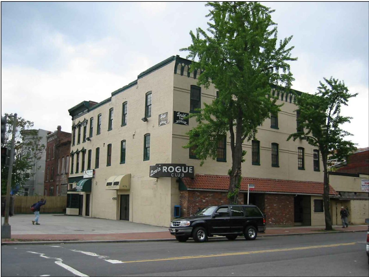
B - VIEW FROM NORTHWEST
