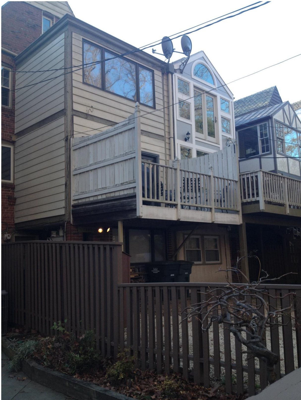
Rear of 1541 44 th showing adjacent structure at 1543 44 th
