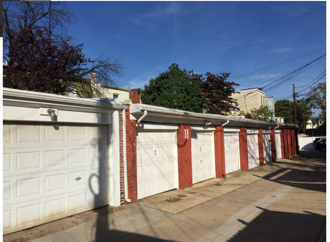
REAR VIEW FROM ALLEY
