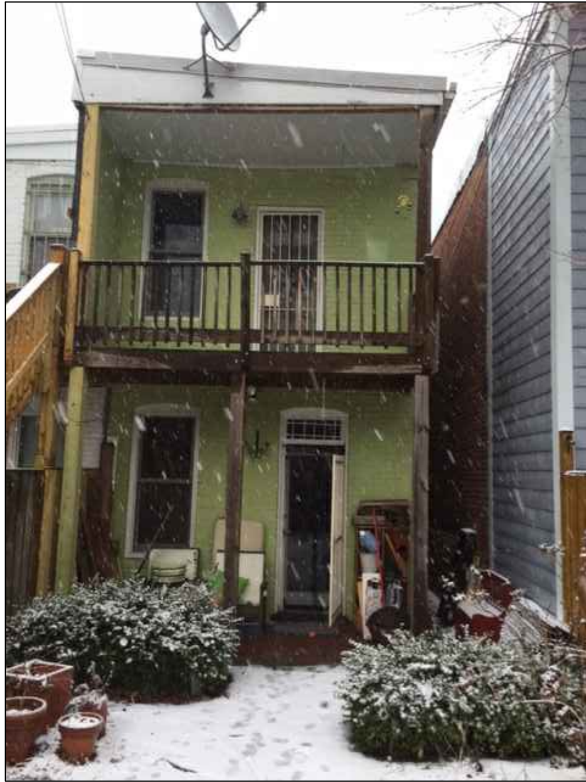
2 230 12TH PLACE NE, VIEW FROM REAR C-4
