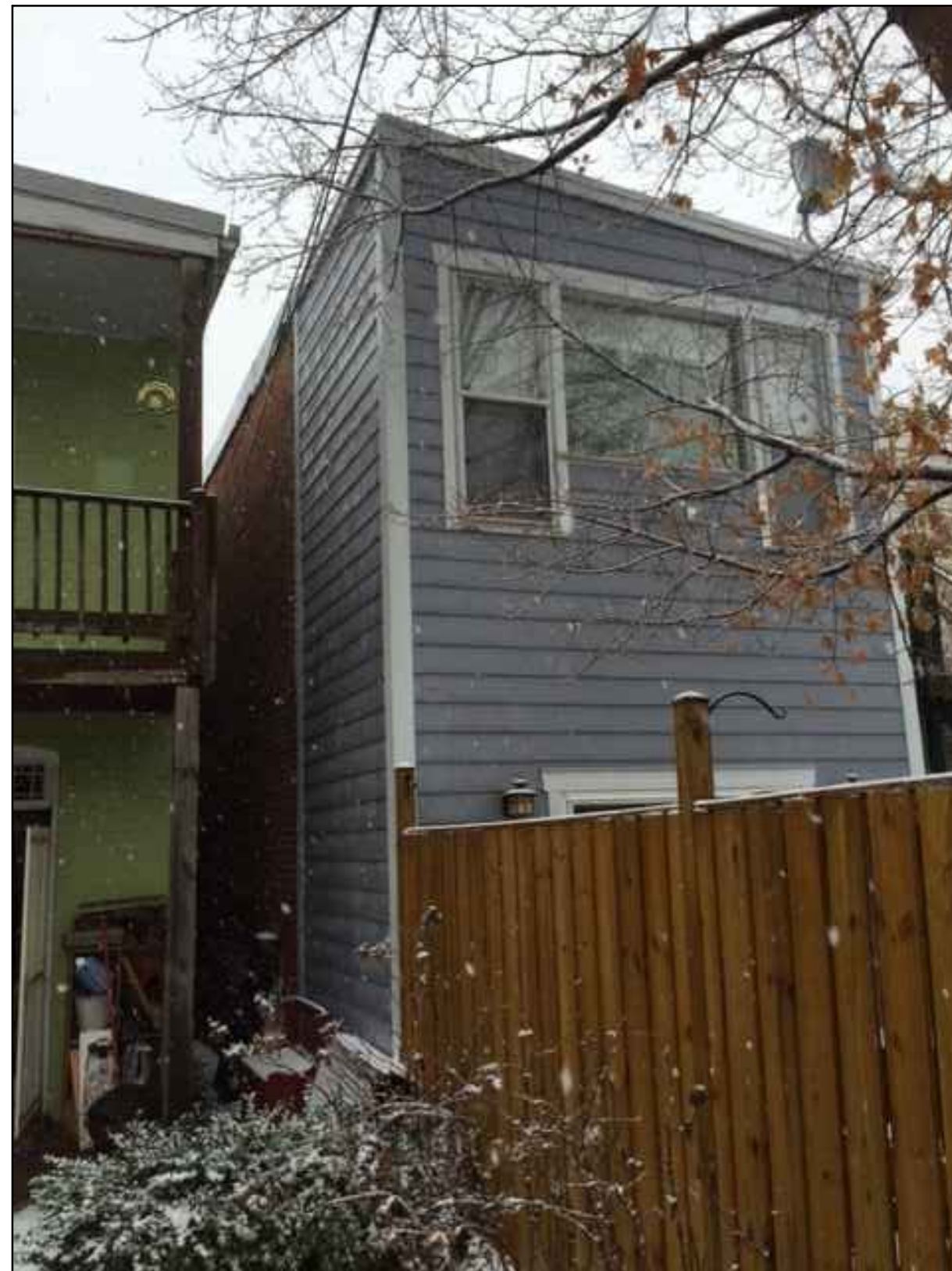
2 VIEW FROM REAR, LOOKING SOUTH C-5
