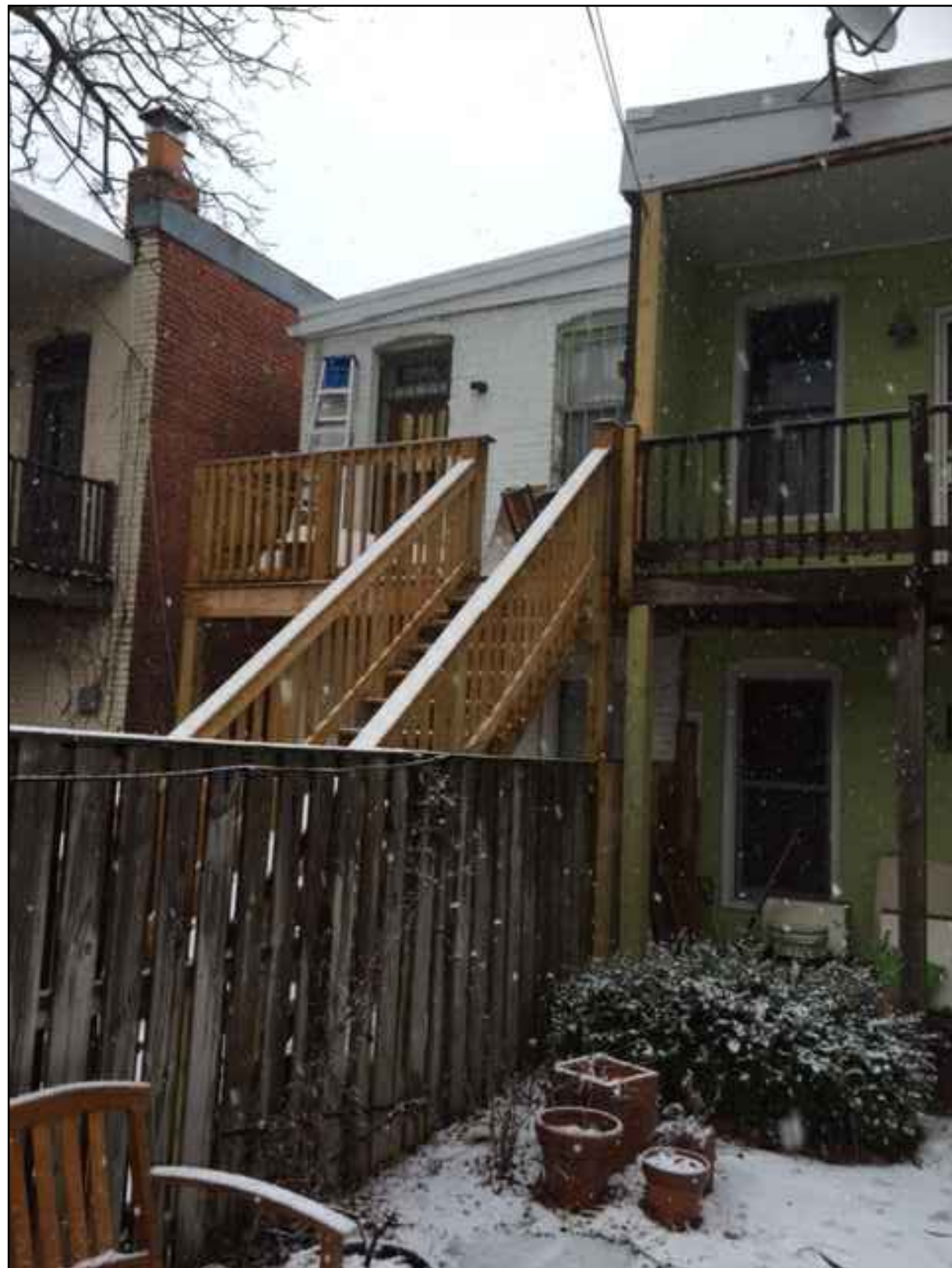
1 VIEW FROM REAR, LOOKING NORTH C-5
