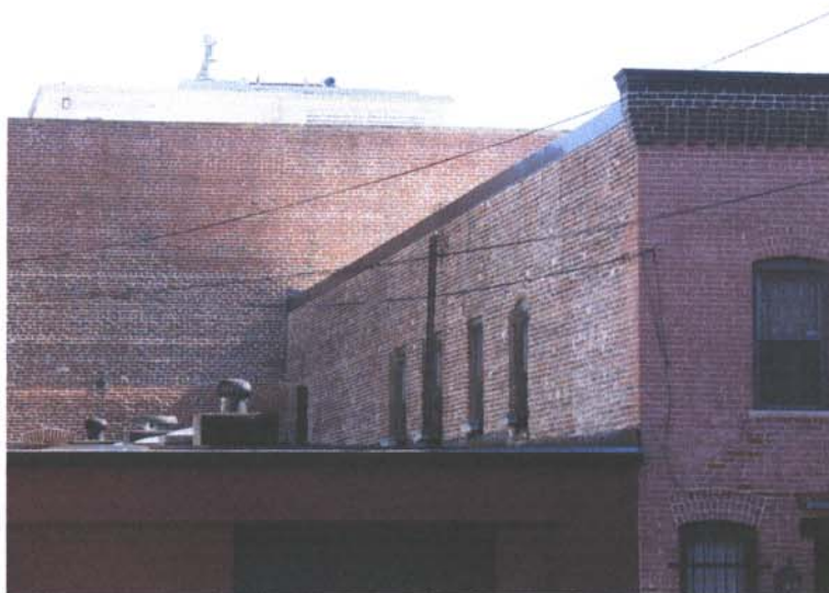
Four windows on 1315 second floor from the outside
