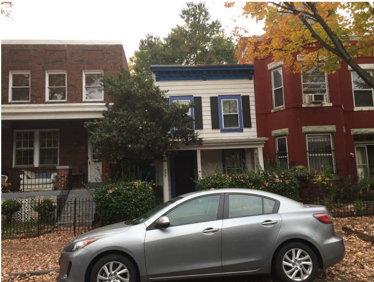
229 10 TH STREET SE- VIEW FROM 10 TH STREET SE
