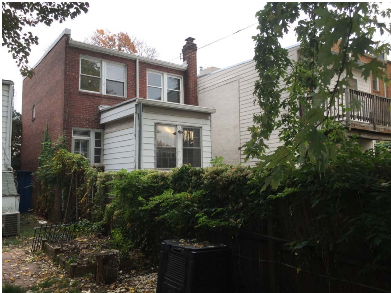
REAR VIEW LOOKING SOUTH
