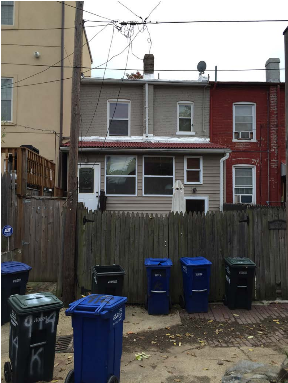
VIEW FROM NORTH
