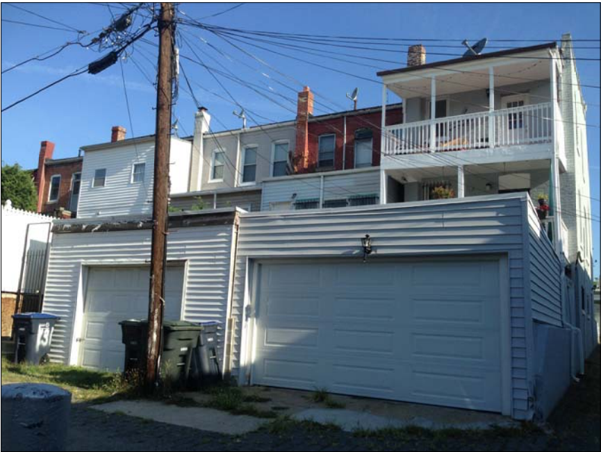
REAR VIEW FROM ALLEY
