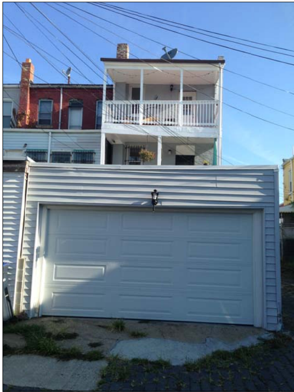
REAR VIEW FROM ALLEY
