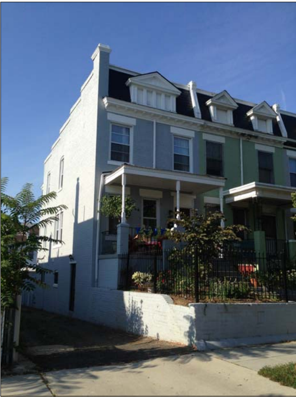
SIDE VIEW FROM U STREET
