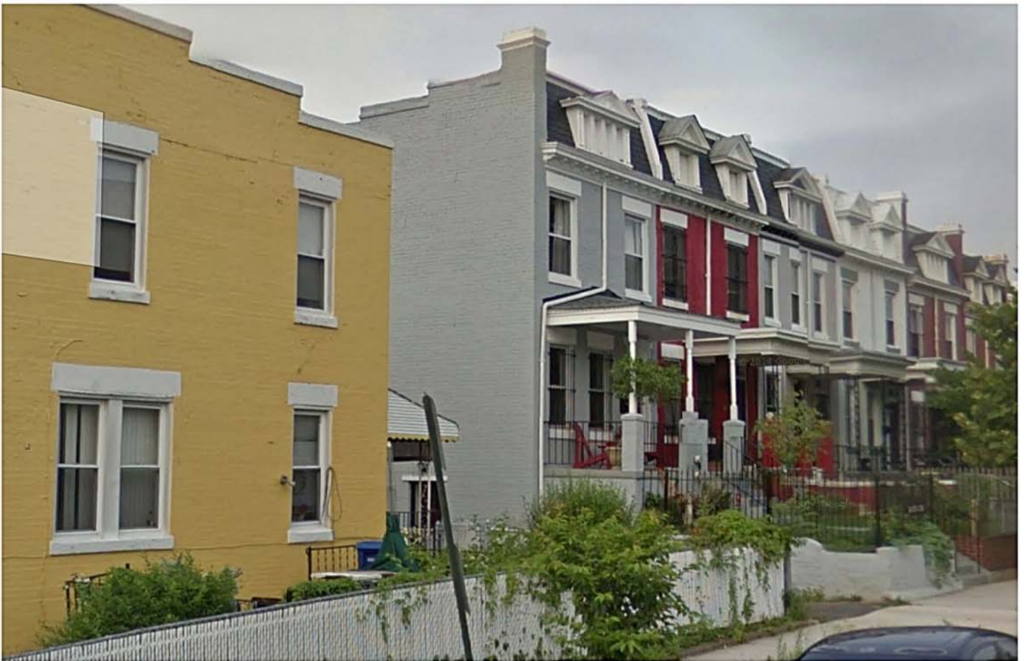
VIEW FROM U STREET
