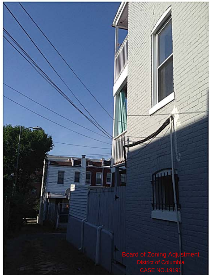
VIEW FROM U STREET LOOKING AT SIDE & REAR ALLIES
