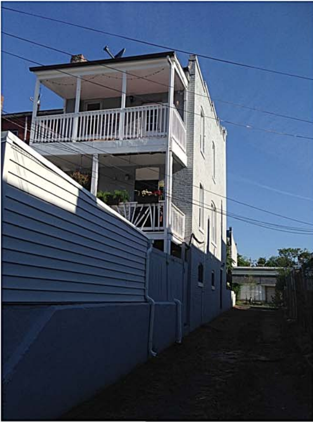
VIEW REAR ALLEY
