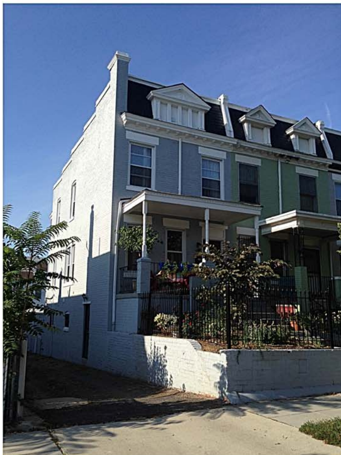
VIEW FROM U STREET
