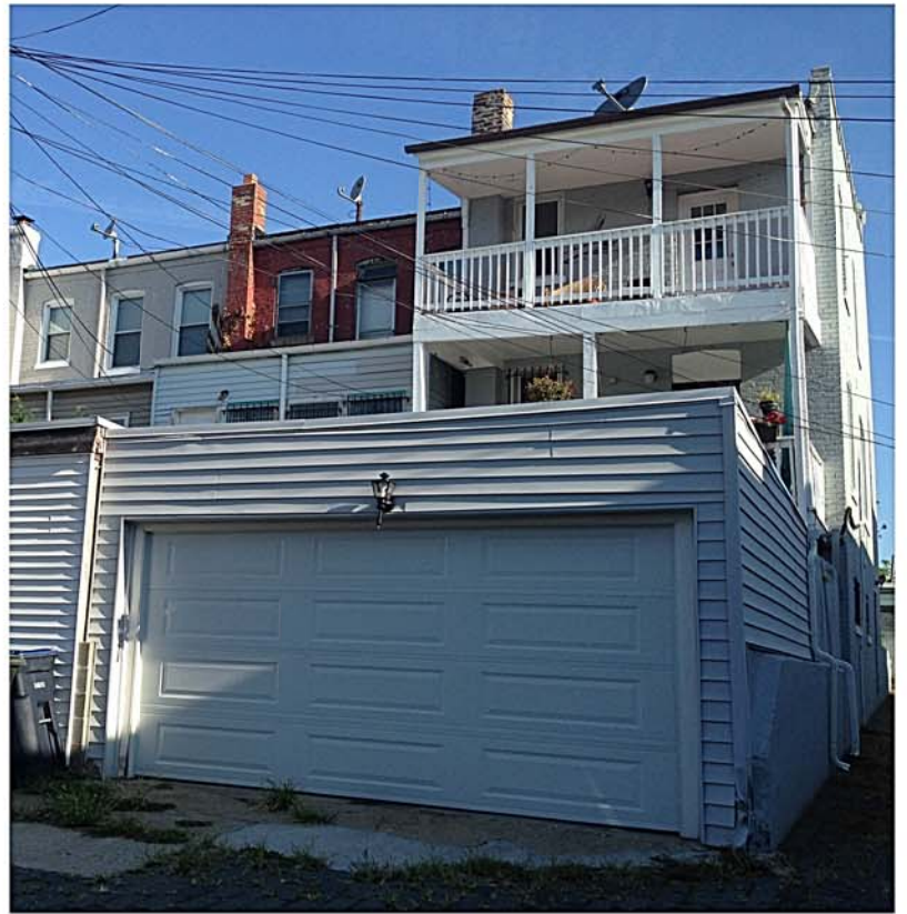
VIEW REAR ALLEY
