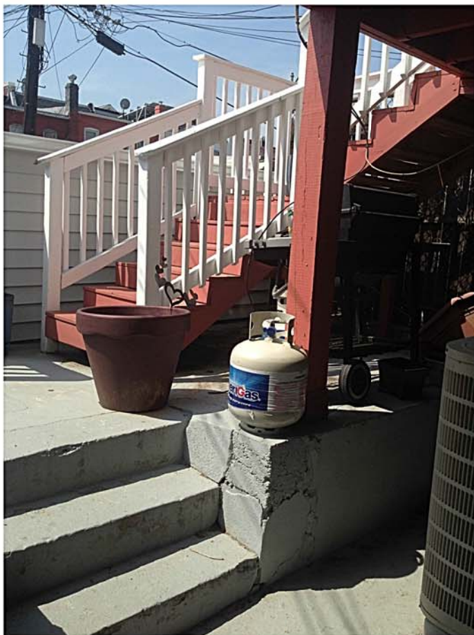
EXISTING STAIR FROM 1ST FLOOR TO CELLAR LEVEL
