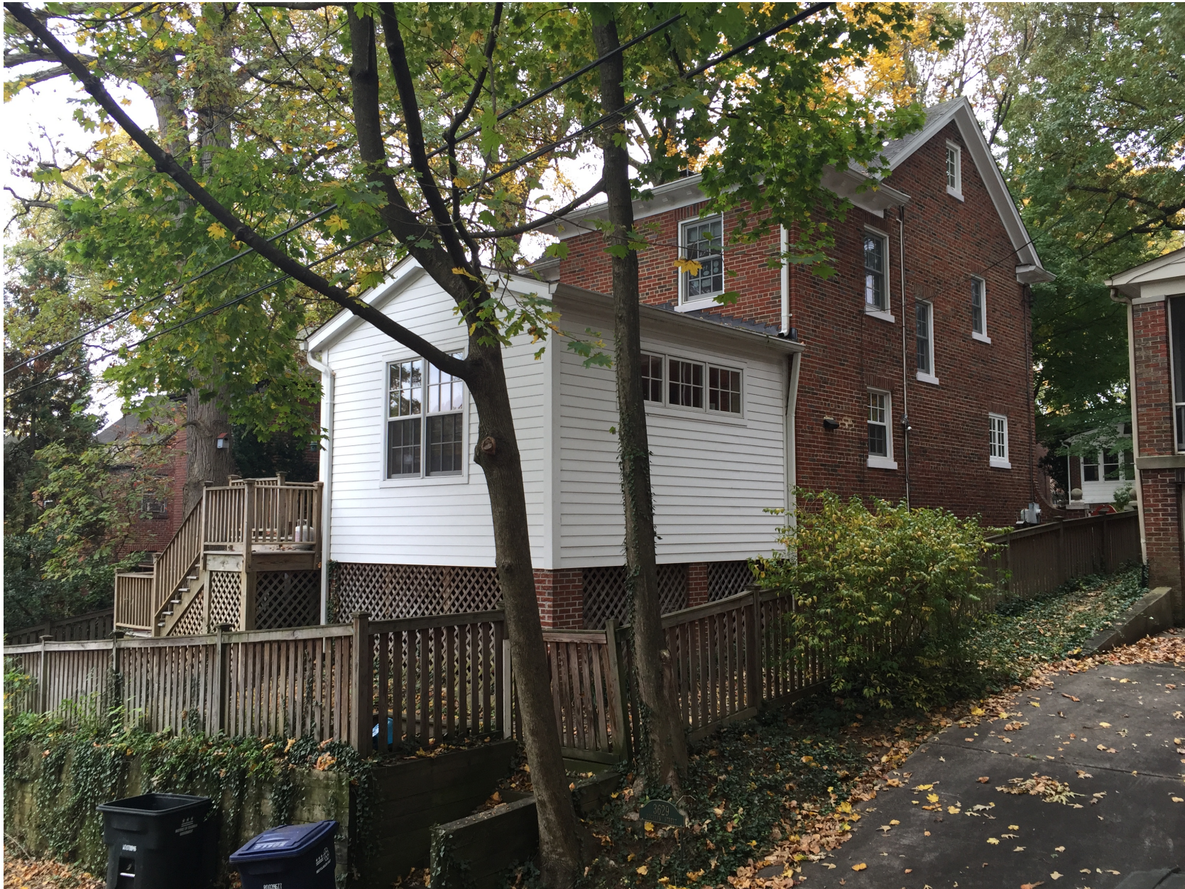
View From Alley East/North Faced
