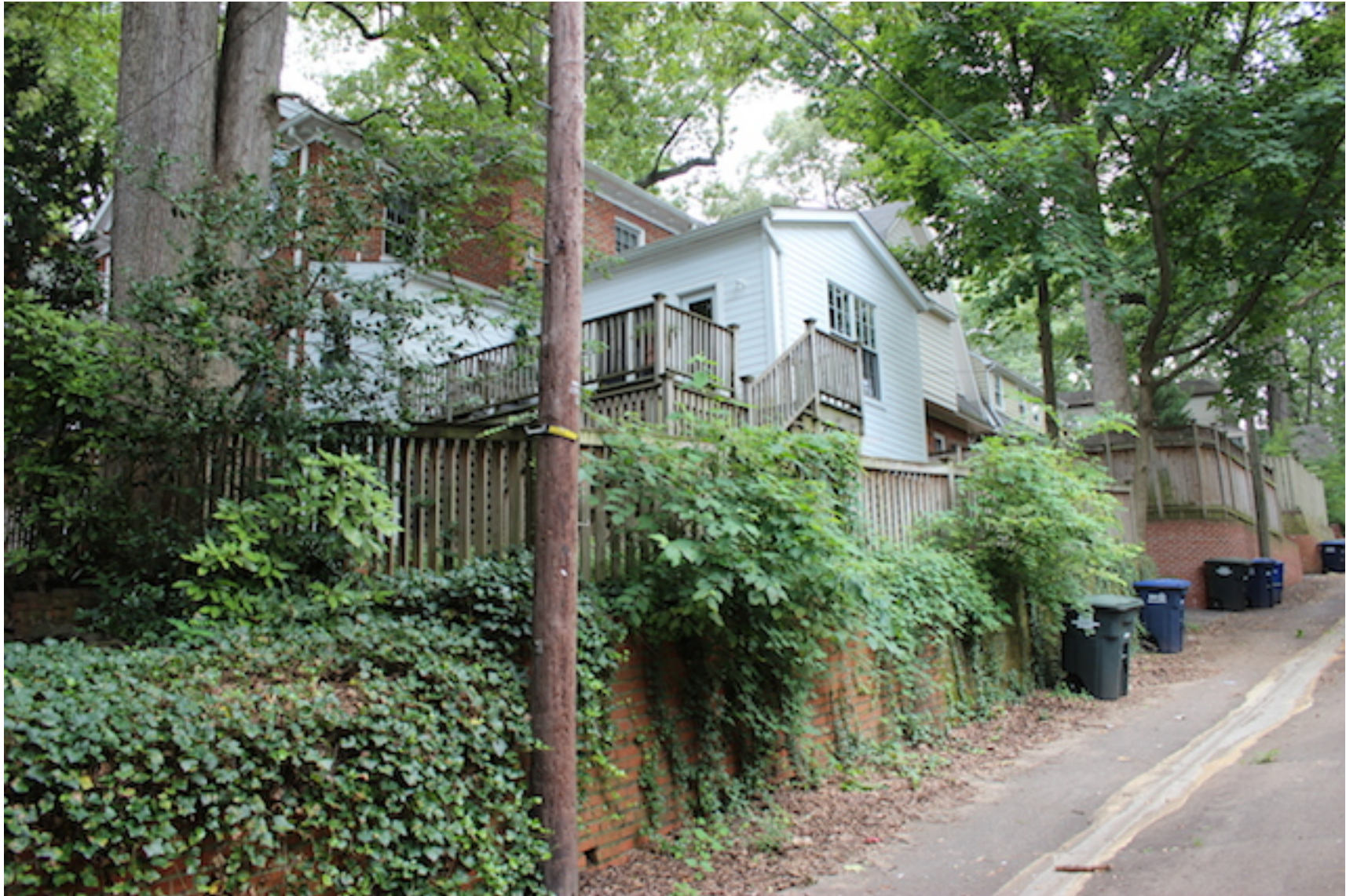
View From Alley West/North Faced
