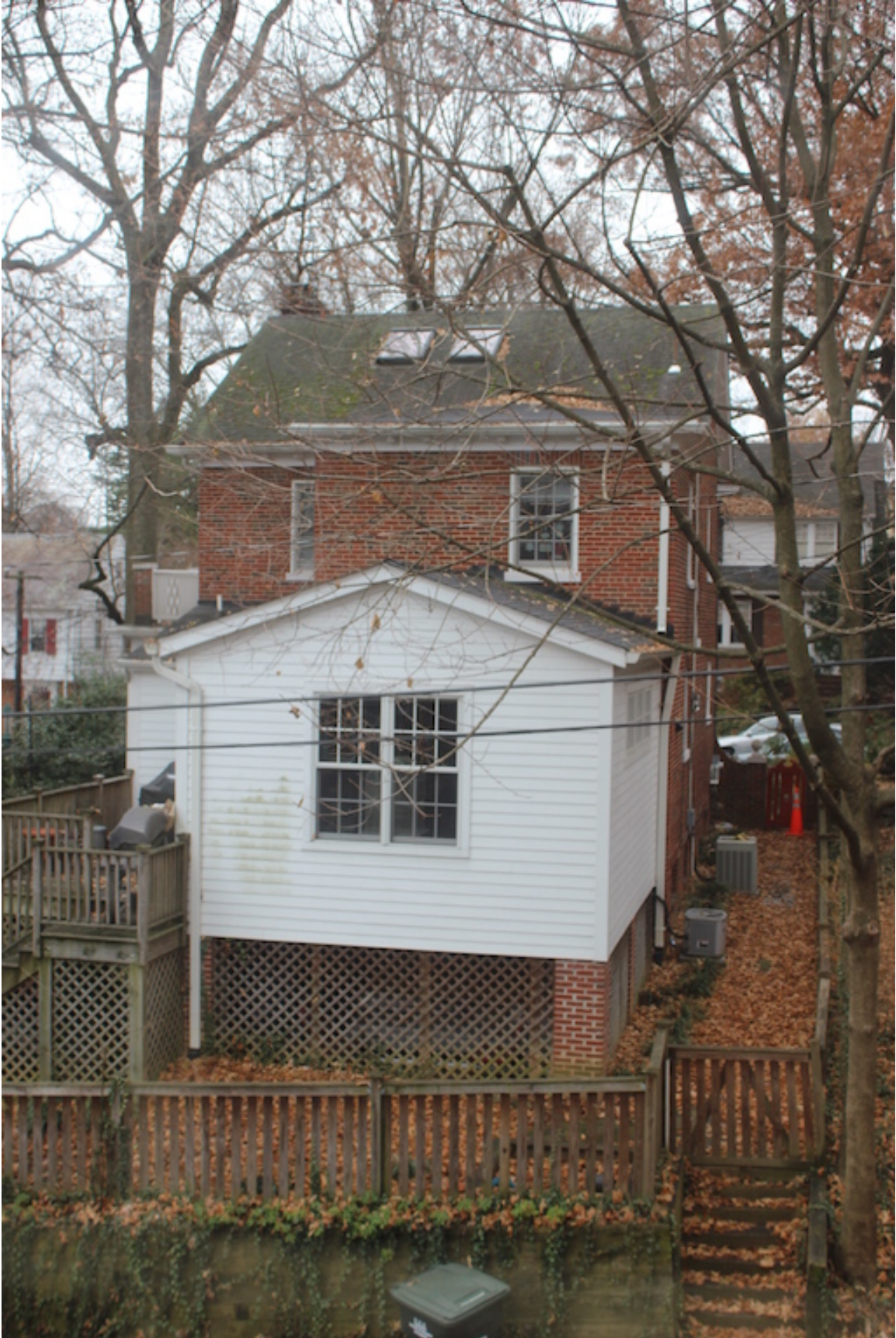
View From Alley (North Facade)
