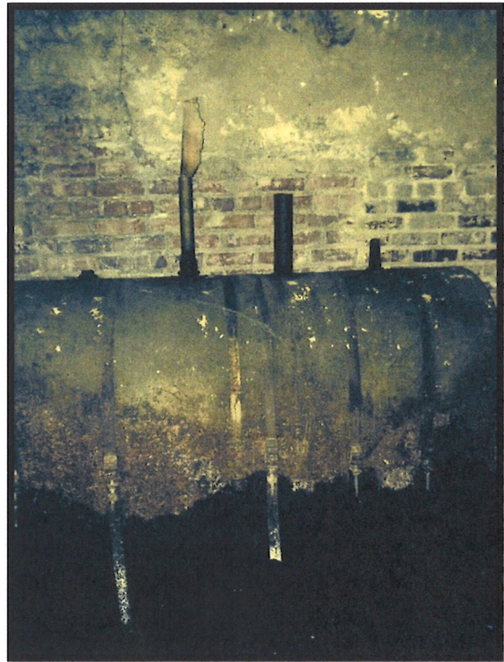
Oil Storage Tank
