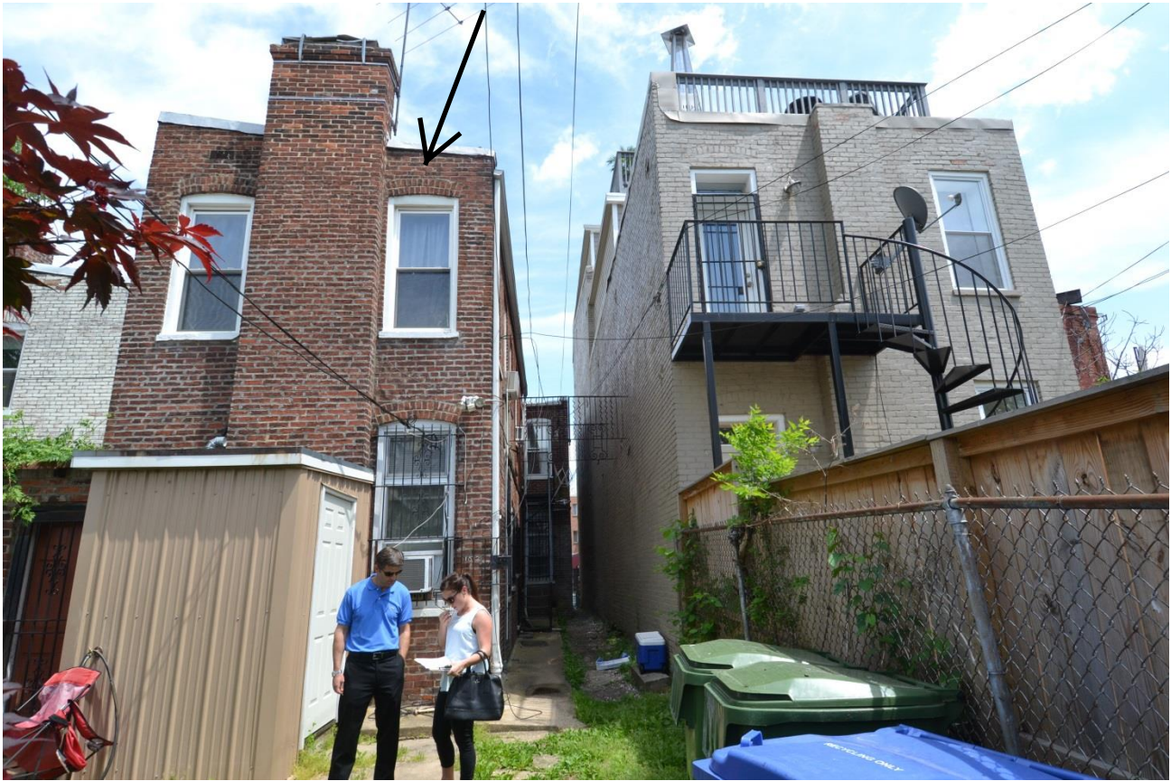
REAR FAÇADE ON PUBLIC ALLEY
