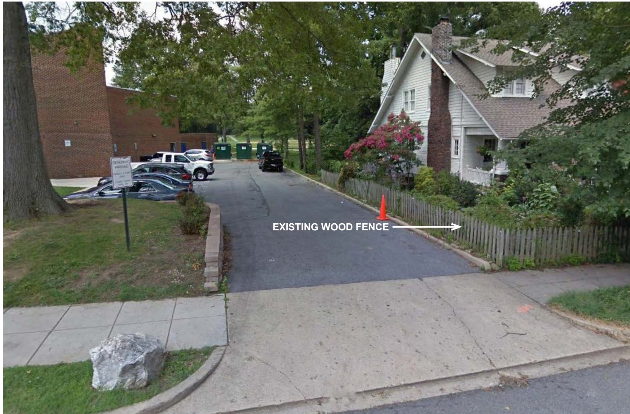
VIEW 5 - EXISTING RESIDENCE FENCE- NEW FENCE TO BE IN-KIND, IN LIEU OF 42" TALL MASONRY WALL
