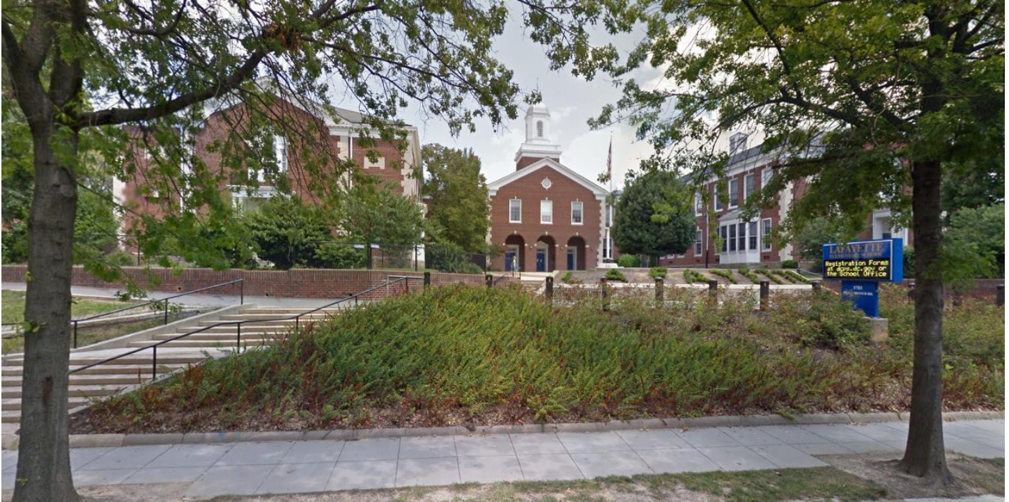
Photo 1: Photo taken looking at front entrance of school (original 1931 building) on 5701 Broad Branch Road NW.
