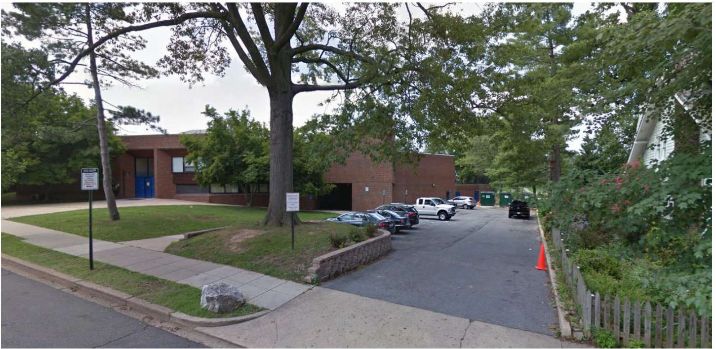
Photo 4: Photo taken looking at the existing school parking lot off Northampton Street NW, which sits adjacent to a private resident at 3307 Northampton Street NW (to the right). The 1970's open-space classroom addition sits to the left of the parking lot.
