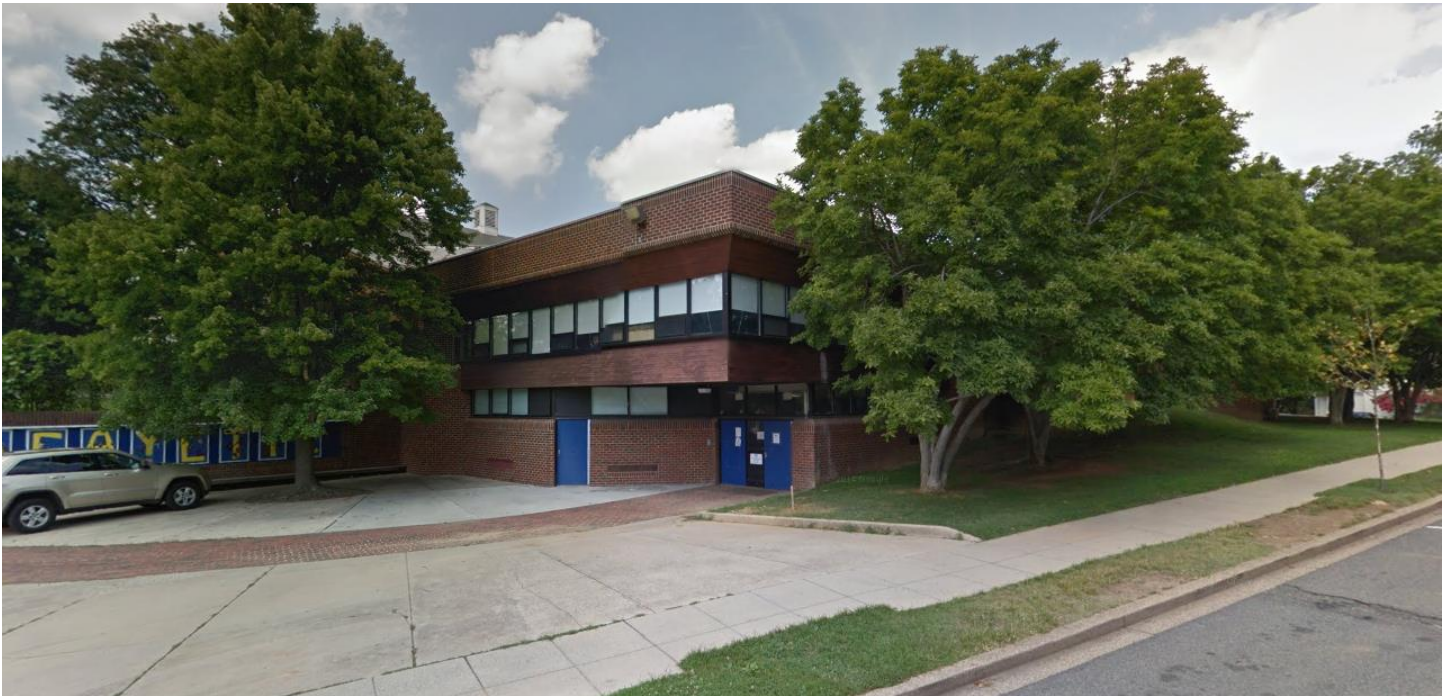
Photo 3: Photo taken looking at 1970's open-space classroom addition from Southampton Street NW, just east of the intersection with Broad Branch Road NW.
