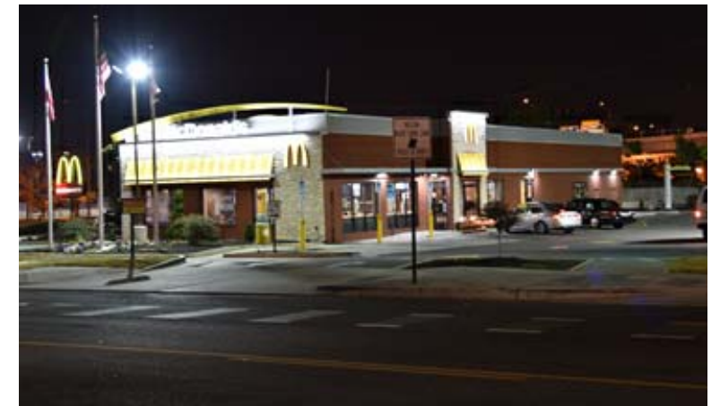
Site Photo 2 - Existing Building
