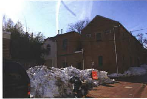
5 EX. SITE - View from NE
