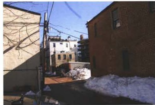
2 EX. SITE - View from NW
