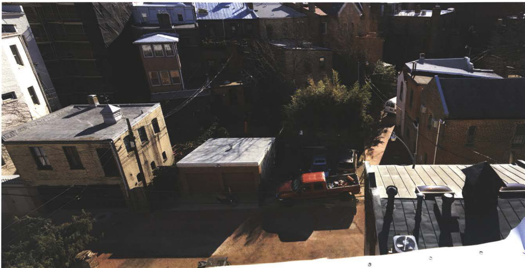
1 EX. SITE - Aerial View from 1310 Q ST
