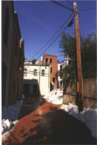
7 EX. SITE - View from SW
