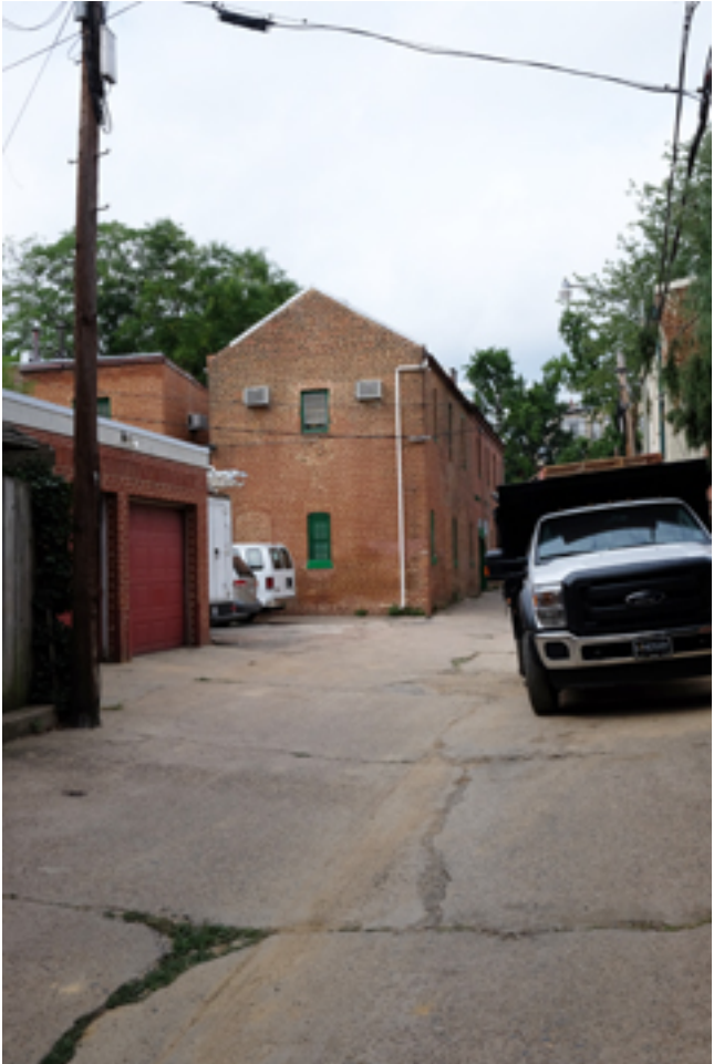
2 EX. SITE - View from NE
