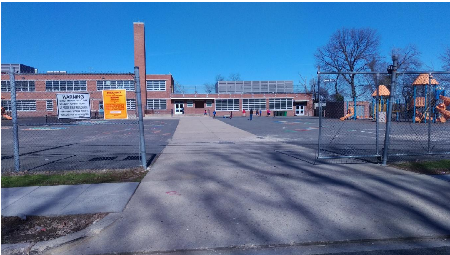
Photo # 4 of 4 - Sign at Morning Drop-off Entrance on C Street, SE (view 2)
