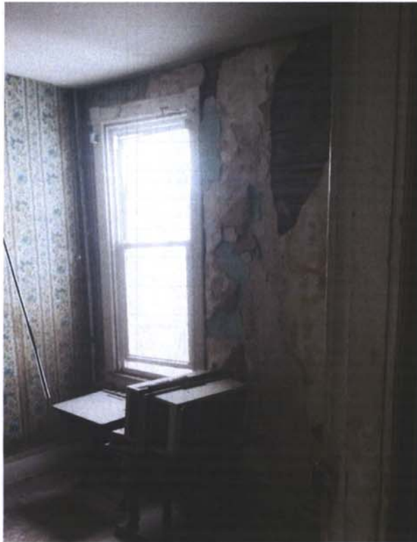
Window on Current Second Floor below Roof Damage (shifting bricks due to water damage)
