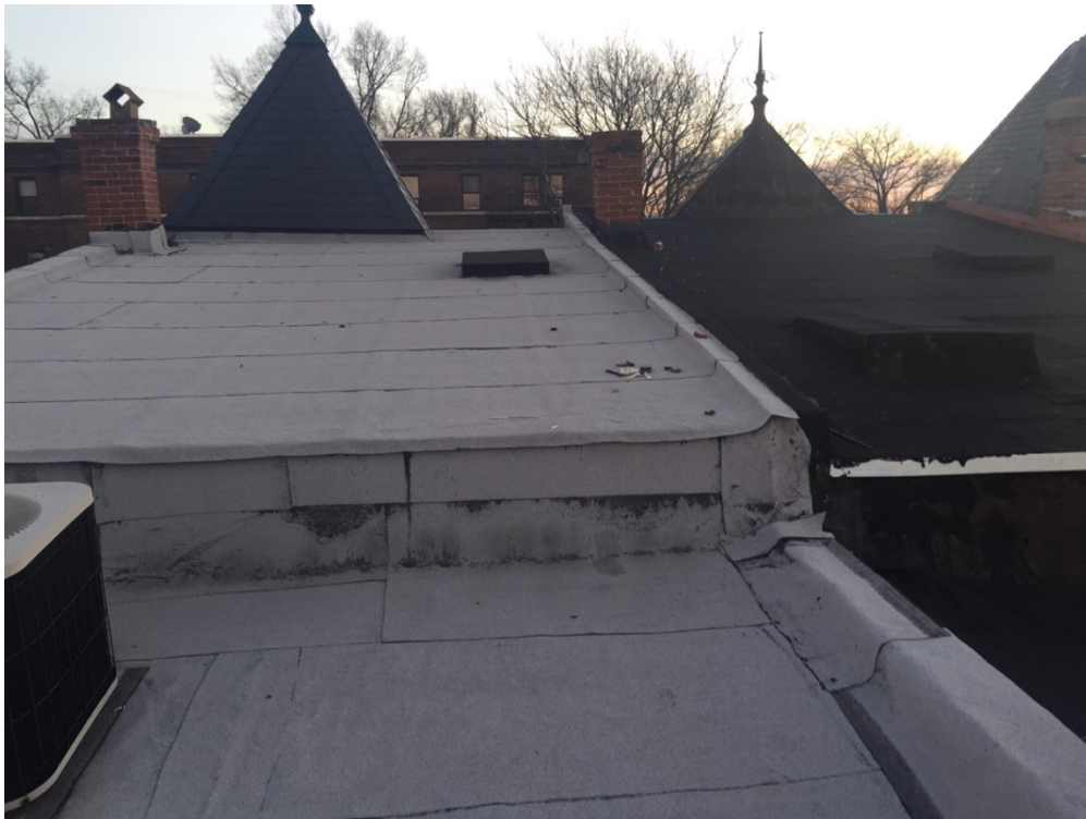
View of Front Roof (white) of 15 U Street NW
