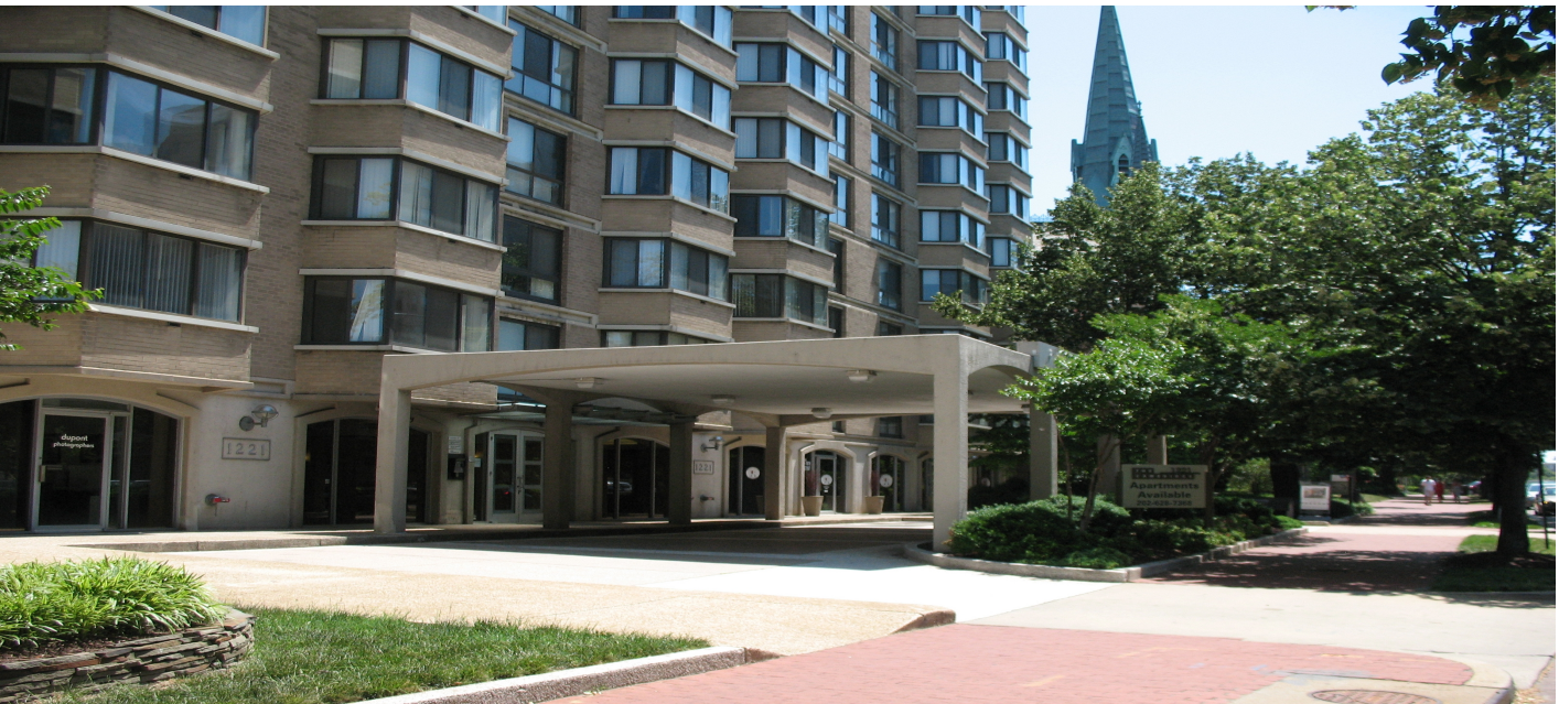
Existing porte-cochere from the west
