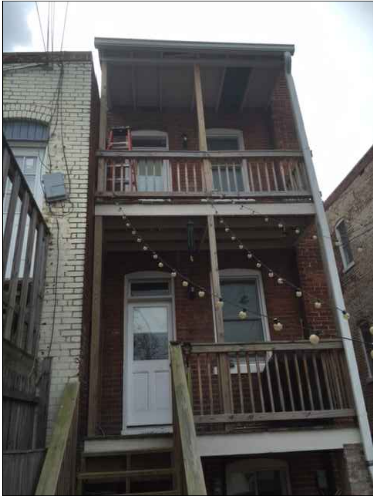
2 REAR OF HOUSE, VIEW FROM REAR YARD C-4
