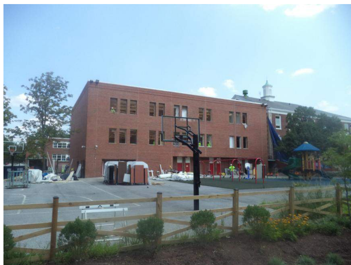
Site Photo (during construction)
