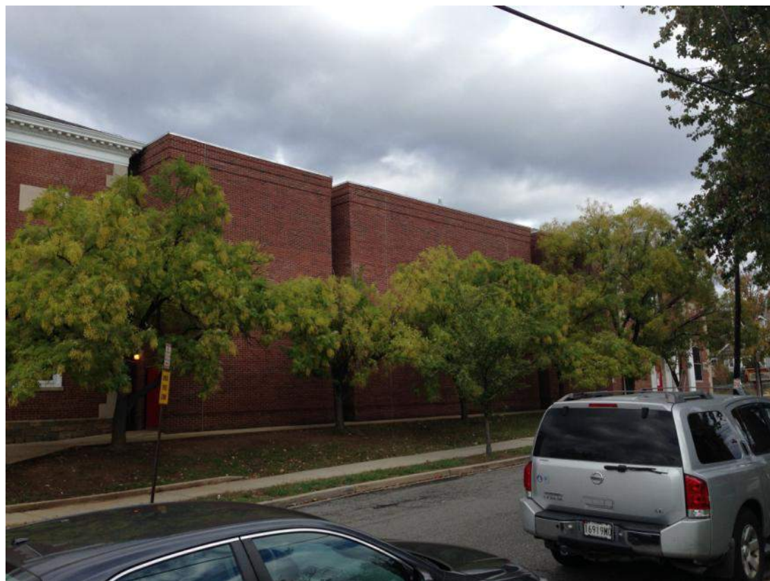
Site Photo (prior to new construction)
