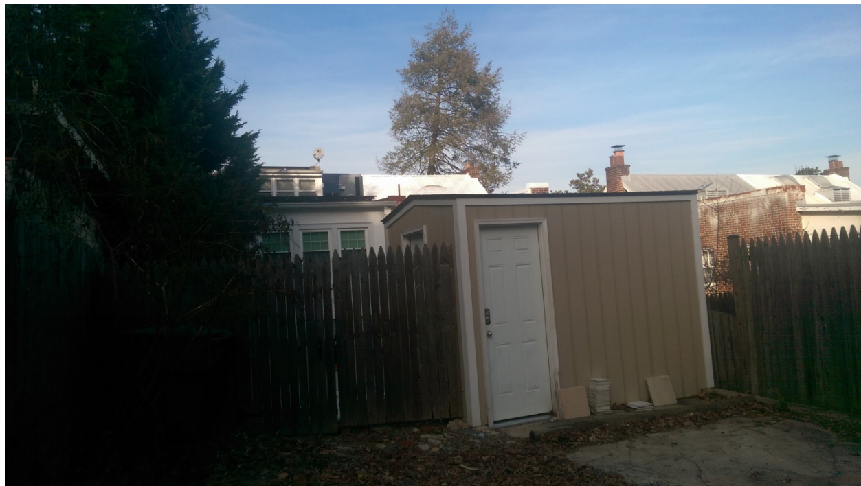
3008 Ordway Rear visibility from alley – Existing 2 nd Floor & Roof
