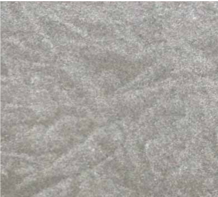
Light-colored honed granite panels at existing exterior columns at ground floor.
