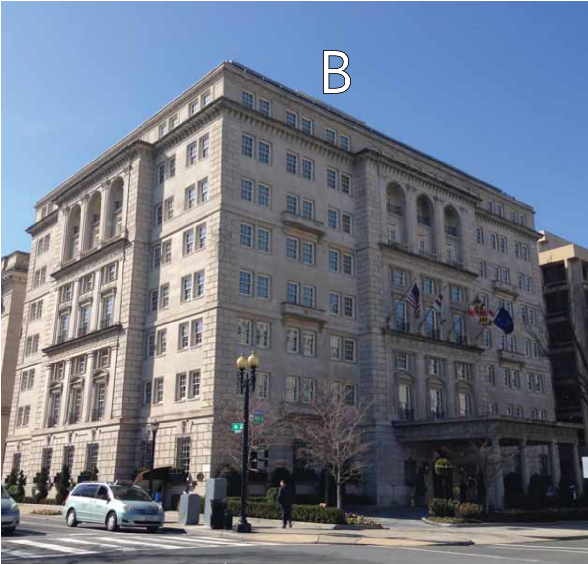
View from intersection of H St NW and 16th St NW looking northwest.
