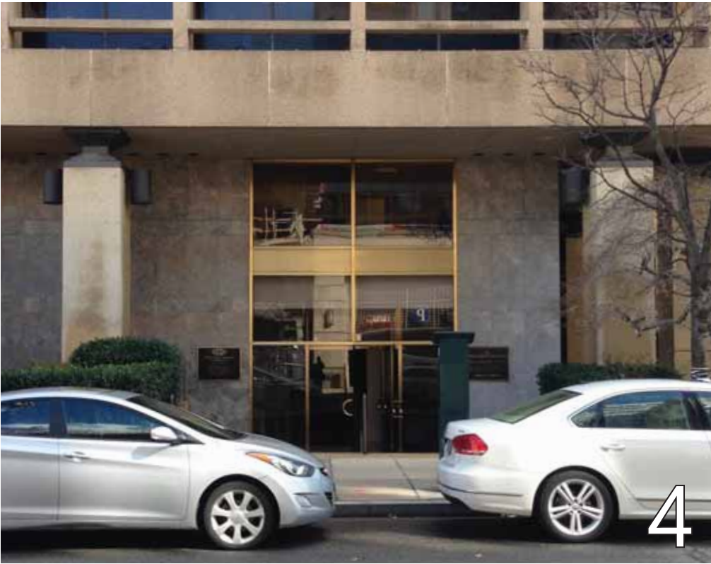
View of MPAA lobby on Eye St NW.
