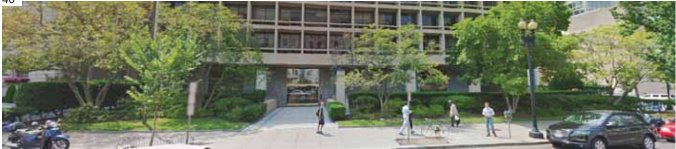
1 View of building entrance from 16th Street NW
