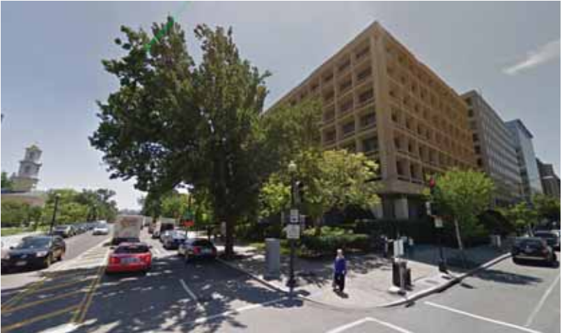
2 View from the intersection of 16th Street NW and Eye Street NW
