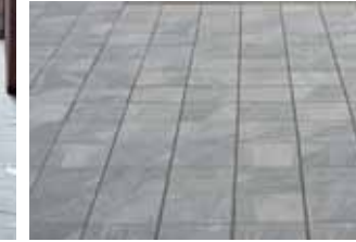
2" STONE PAVING on 1" sand setting bed and 4" concrete base over 4" of aggregate
