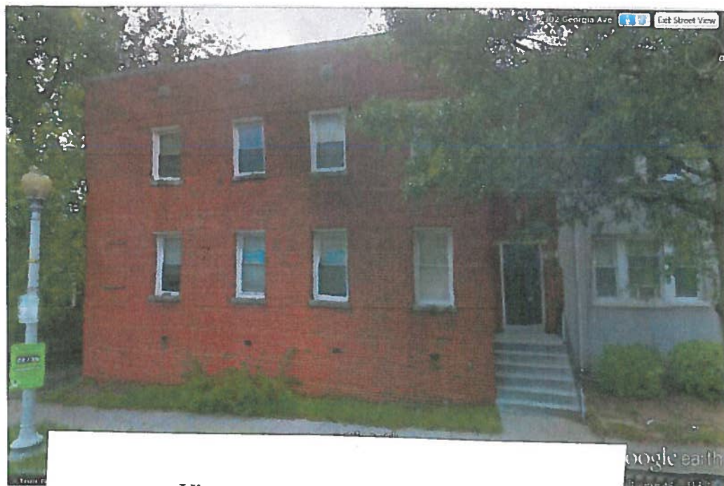
View of the front of the Subject Building
