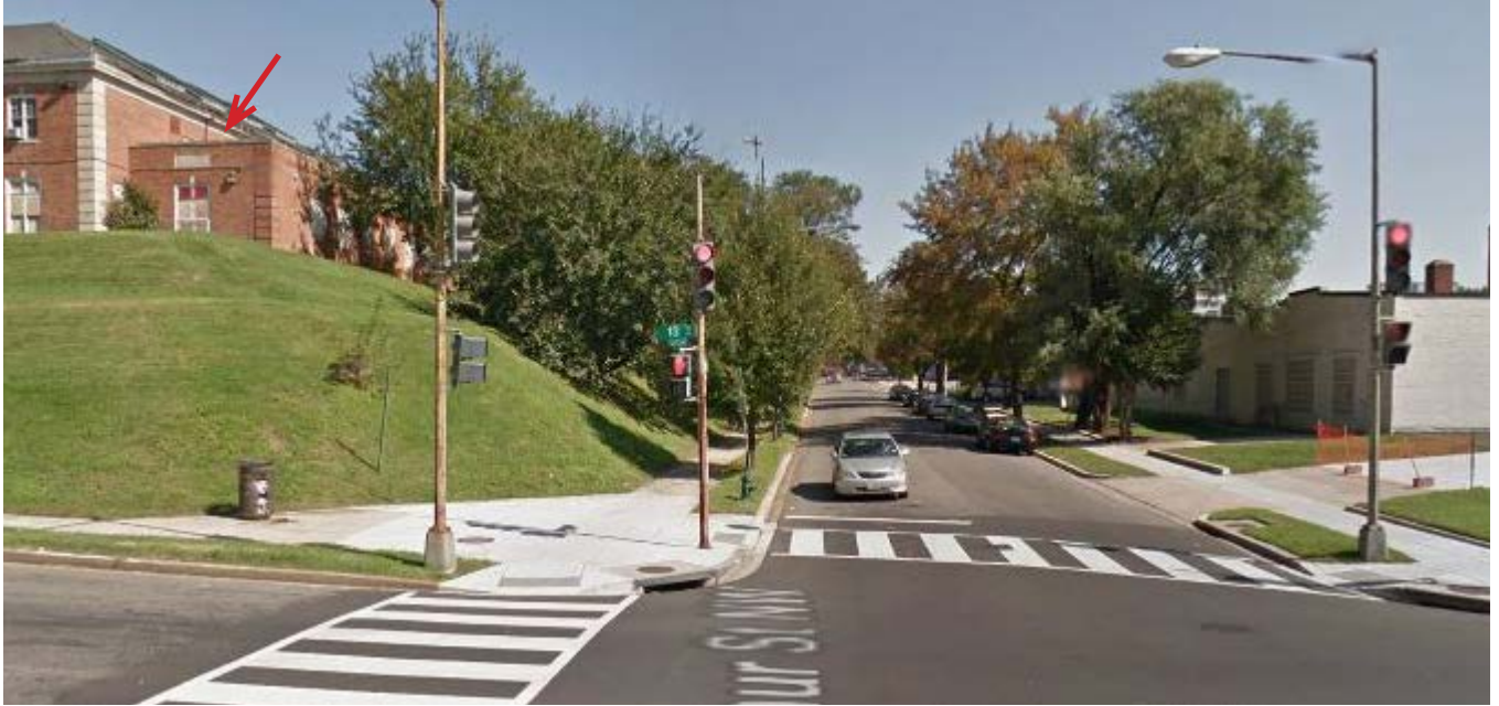
FIGURE 7: The intersection of 13th Street NW and Upshur Street NW, looking east. The gymnasium can be seen on top of the stepped terraces of the Property. The red arrow indicates the roof top area for which the Applicant is requesting a special exception.
