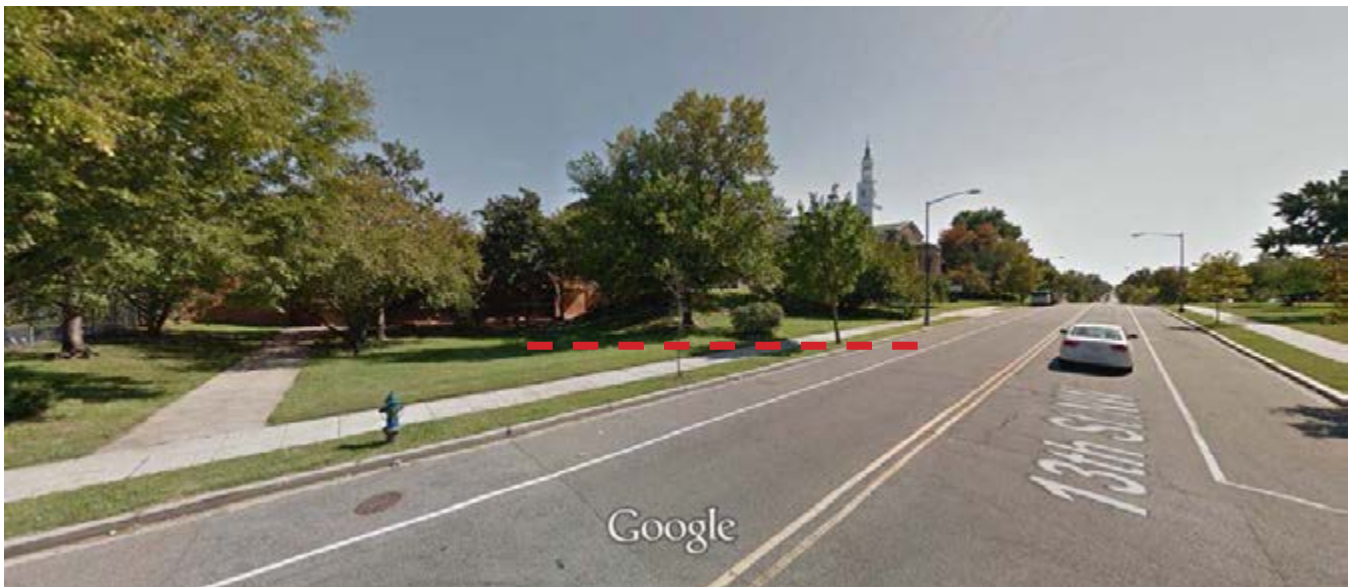
FIGURE 3: View from 13th Street NW adjacent to area where new bus drop off and parking lot is proposed. Red dashed line indicates location where existing topography of the site begins to slope steeply upward.
