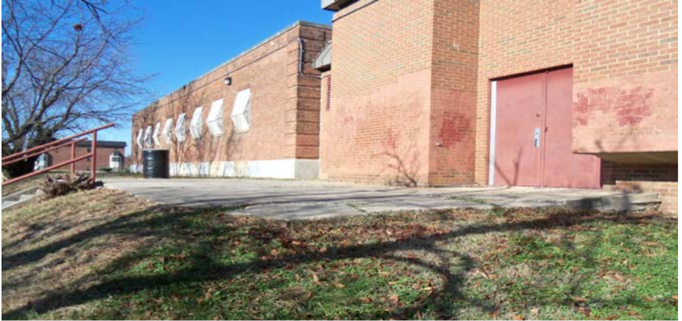
FIGURE 9: View of the south facade of the Property. The red arrow indicates the roof top area for which the Applicant is requesting a special exception.
