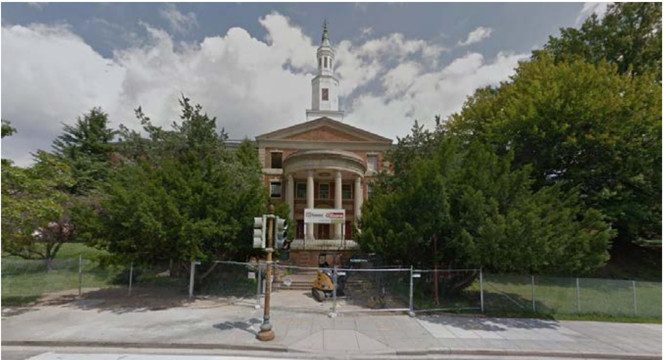
FIGURE 6: Existing conditions view of the main entrance to Roosevelt High School, from 13th Street NW.
