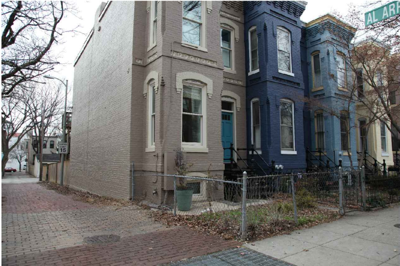
6. VIEW FROM 11th STREET
