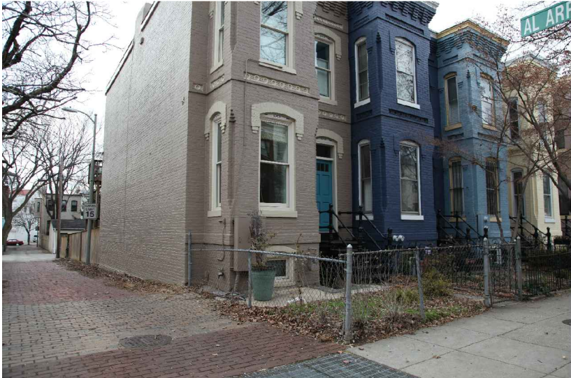
6. VIEW FROM 11th STREET
