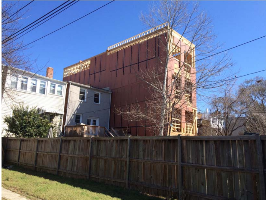
Image 10, depicts similar construction / conversion of row house in the Bloomingdale neighborhood at 42 W Street NW, (one block north of subject property).
