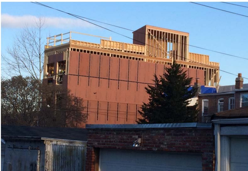
Image 9, depicts similar construction / conversion of row house in the Bloomingdale neighborhood at 42 W Street NW, (one block north of subject property).
