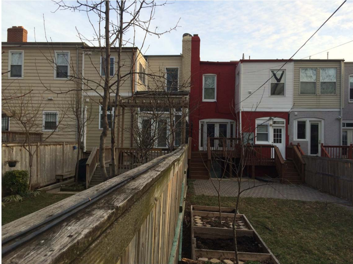
Image 6, depicts the rear of the subject property (in red and white, before demolition). To the left is 65 V Street NW and to the right is, 69 V Street NW.
