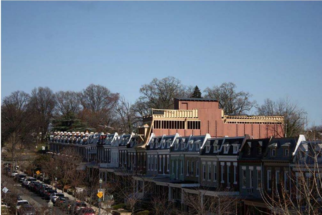
Image 8, depicts similar construction / conversion of row house in the Bloomingdale neighborhood at 42 W Street NW, (one block north of subject property).
