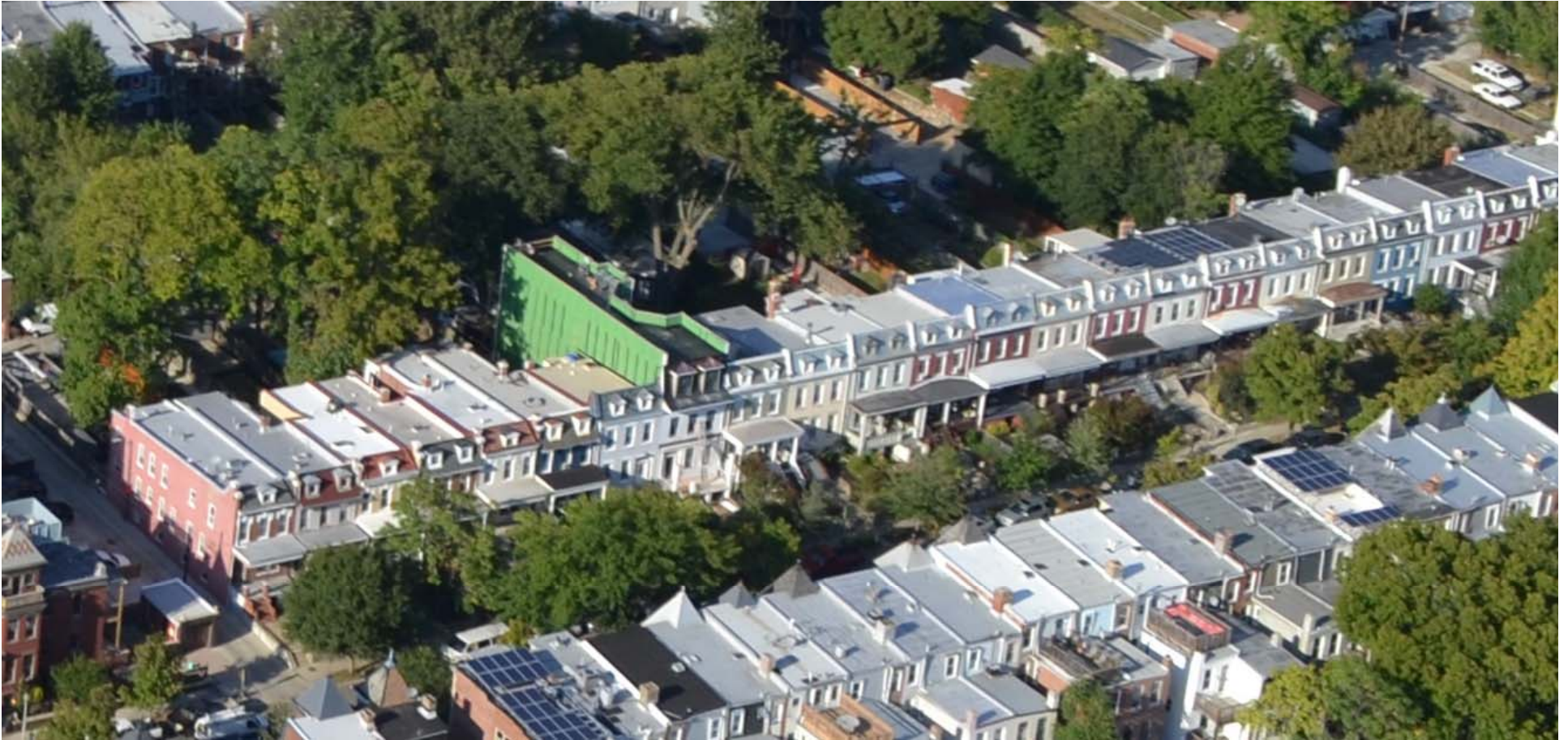
Unit block of V Street NW, 67 V shown in green.
