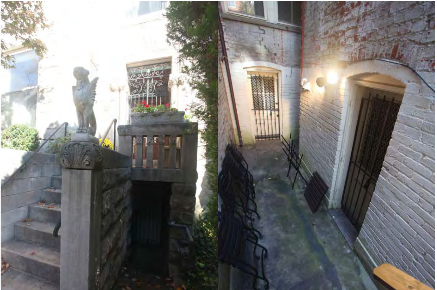
Existing front entrance to basement
