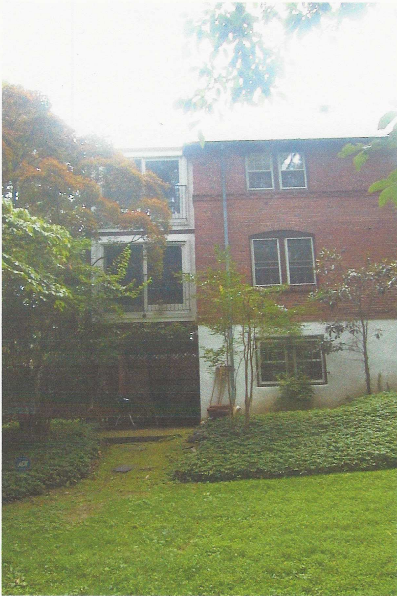
PHOTO 4 VIEW OF EAST SIDE OF HOUSE (PHOTO TAKEN FROM ARCHBOLD GLOVER PARK)
