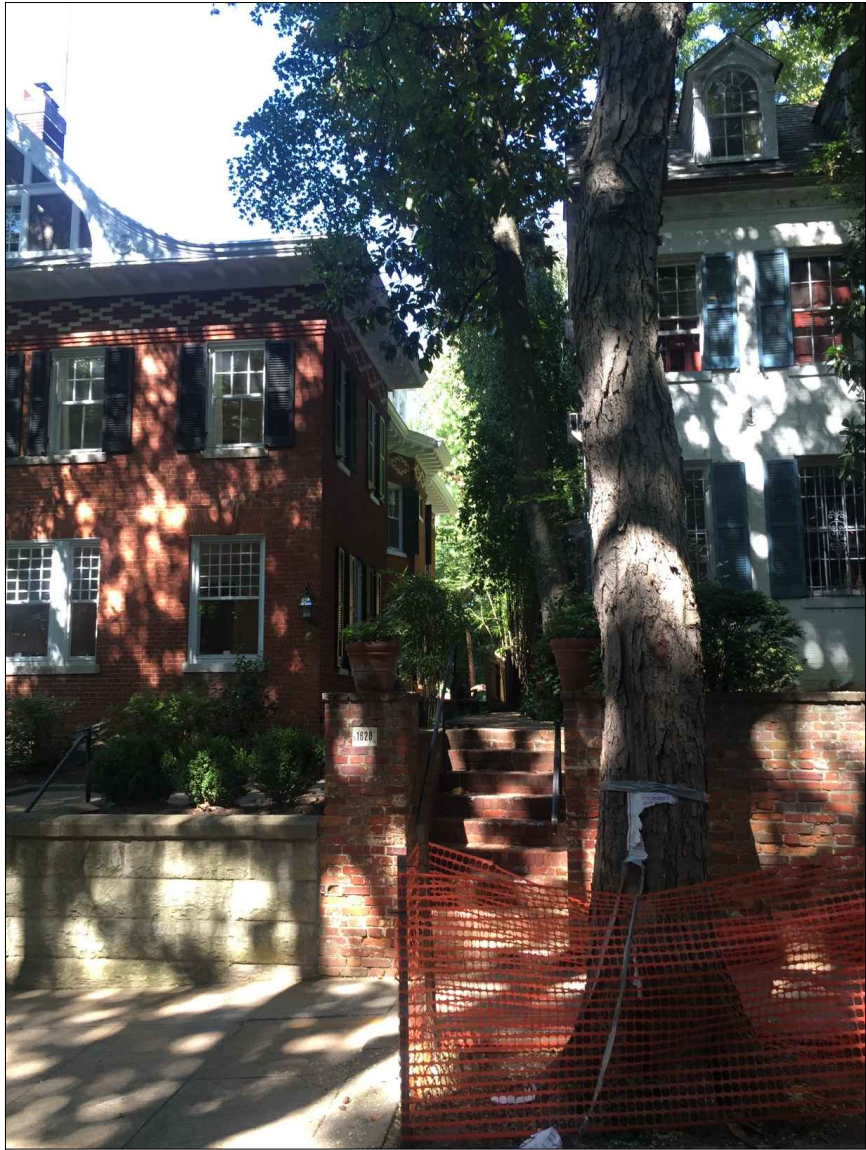
1 VIEW FROM 29TH STREET
