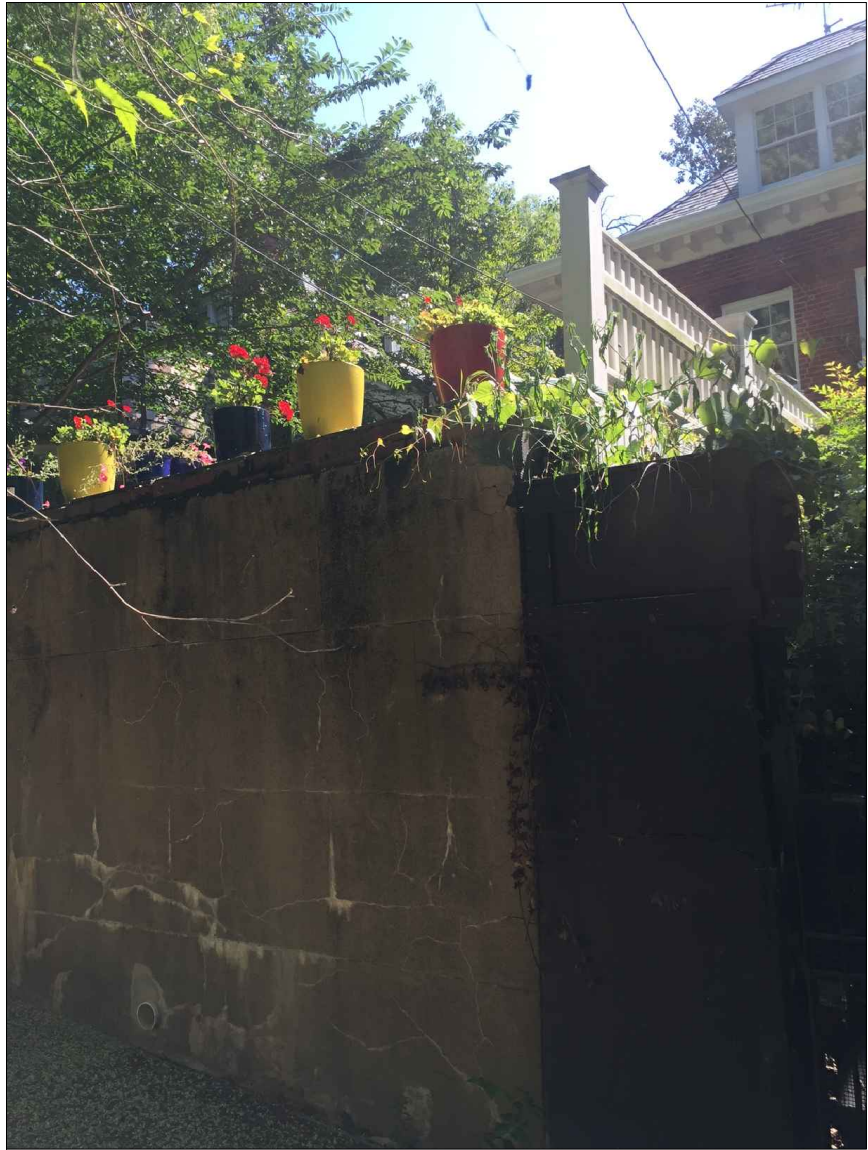
3 VIEW FROM REAR ALLEY
