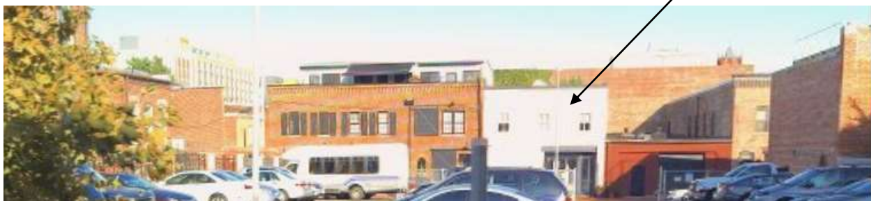
Street View with Adjacent Properties
