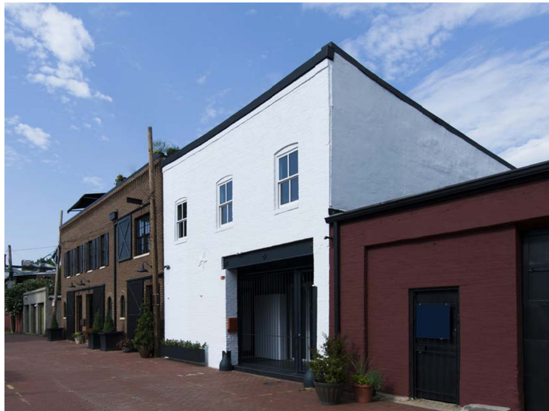
1 1319 NAYLOR CT ALLEY FACADE
