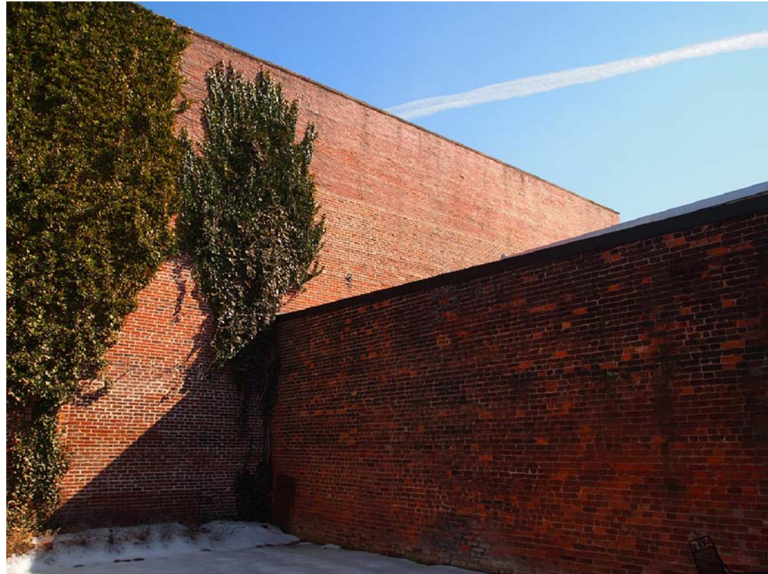
2 REAR YARD SITE WALLS
