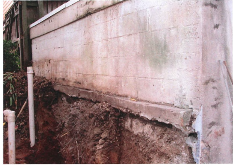
Garage construction 1120 Park St. NE affecting wall of garage at 1118 Park St. NE. Photos June 7 and June 13
