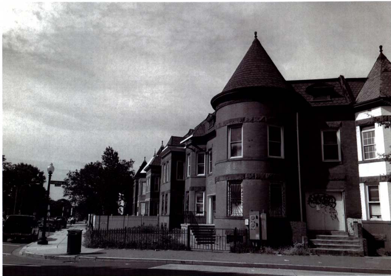
EXISTING CONDITIONS PHOTO - FLORIDA AVE ELEVATION
