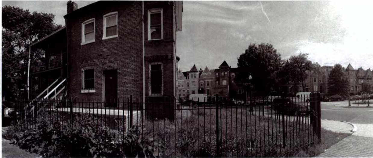
EXISTING CONDITIONS PHOTO - REAR ALLEY ELEVATION
