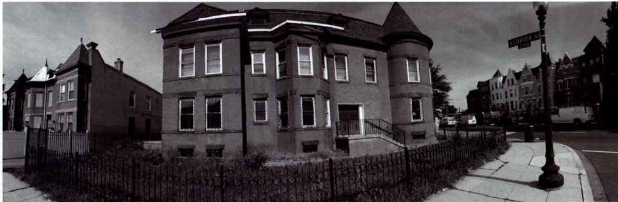
EXISTING CONDITIONS PHOTO - 3RD ST ELEVATION
