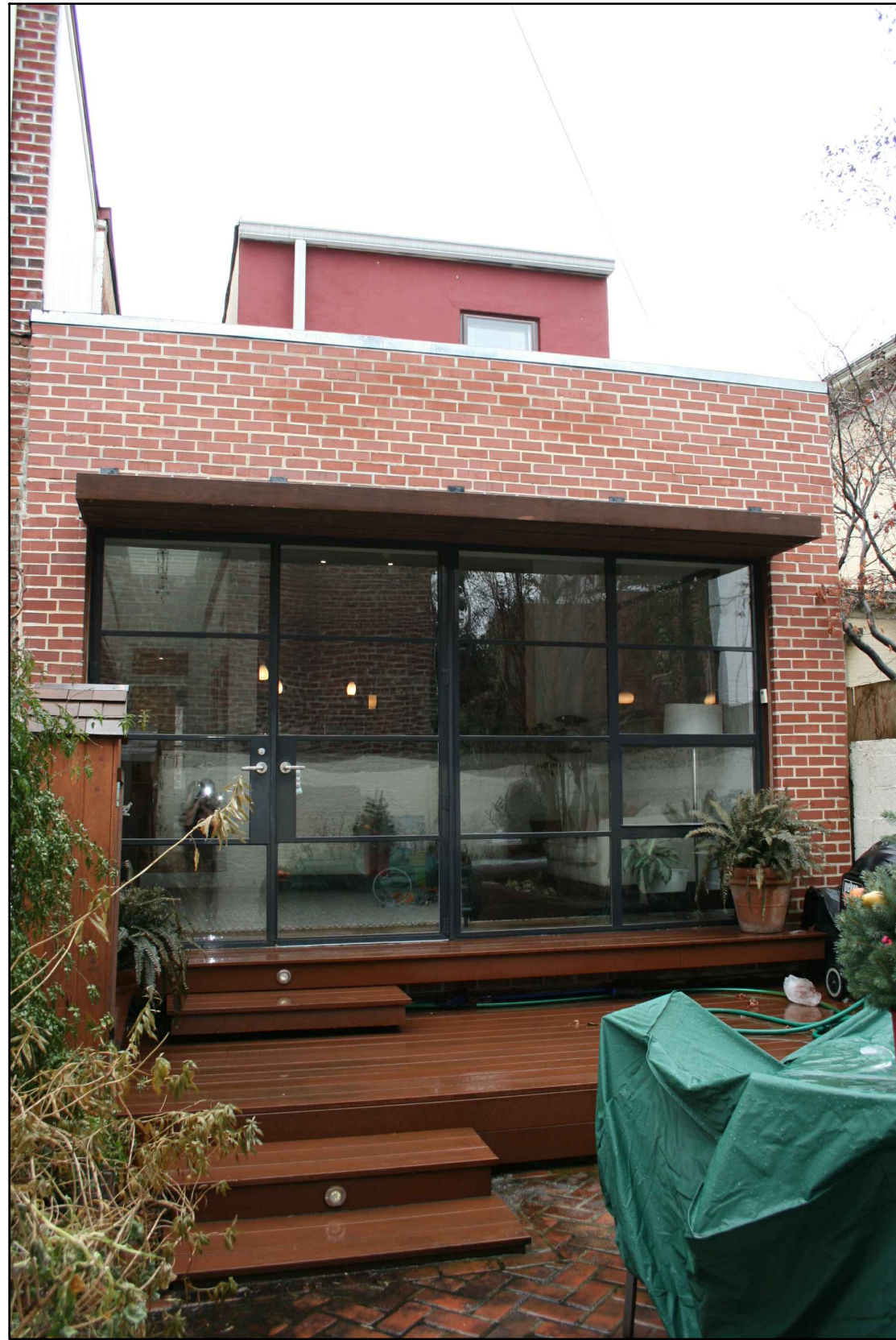
2 C-4 602 A ST NE, VIEW FROM REAR
