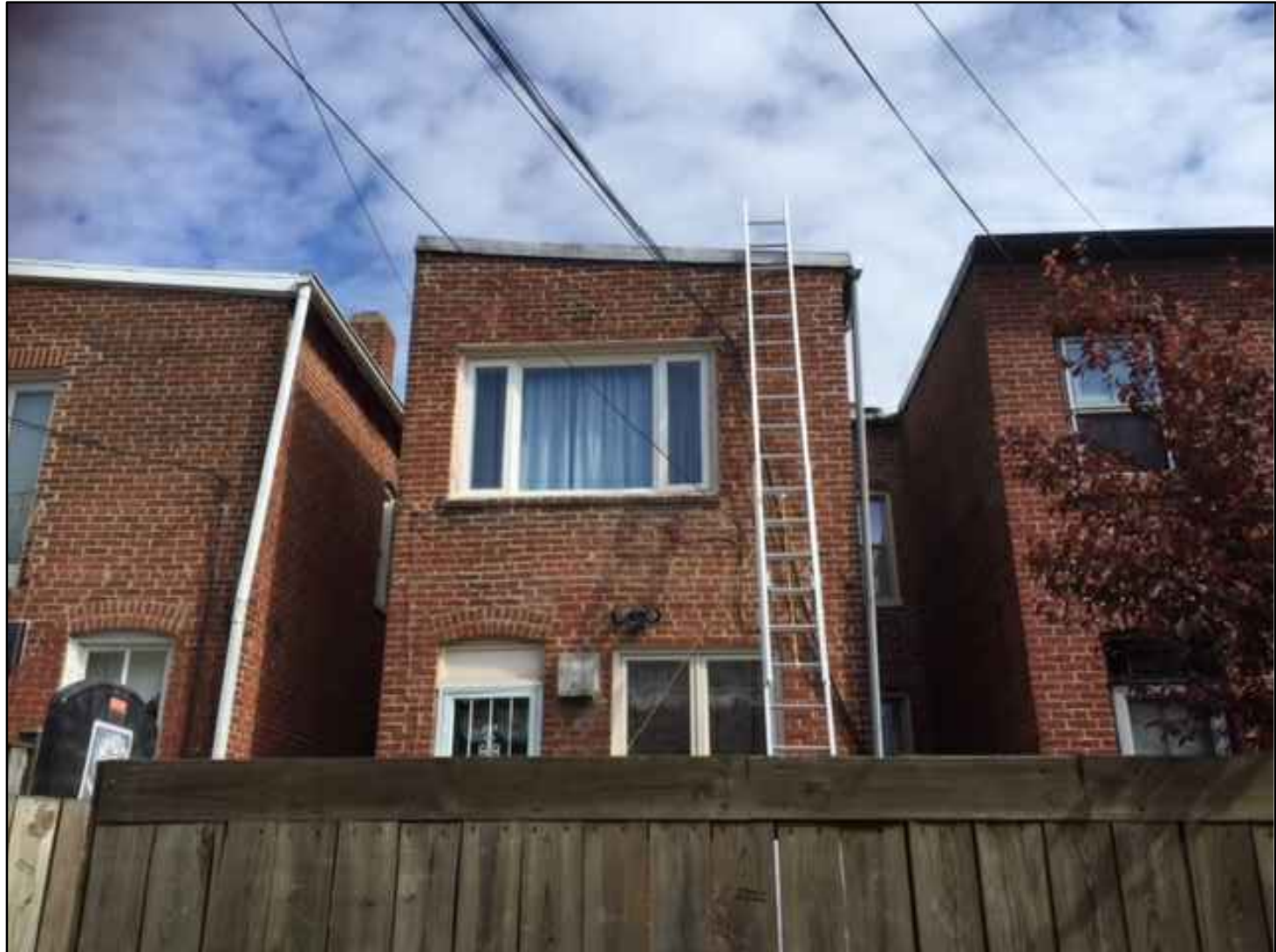
2 REAR OF HOUSE, VIEW FROM ALLEY C-4
