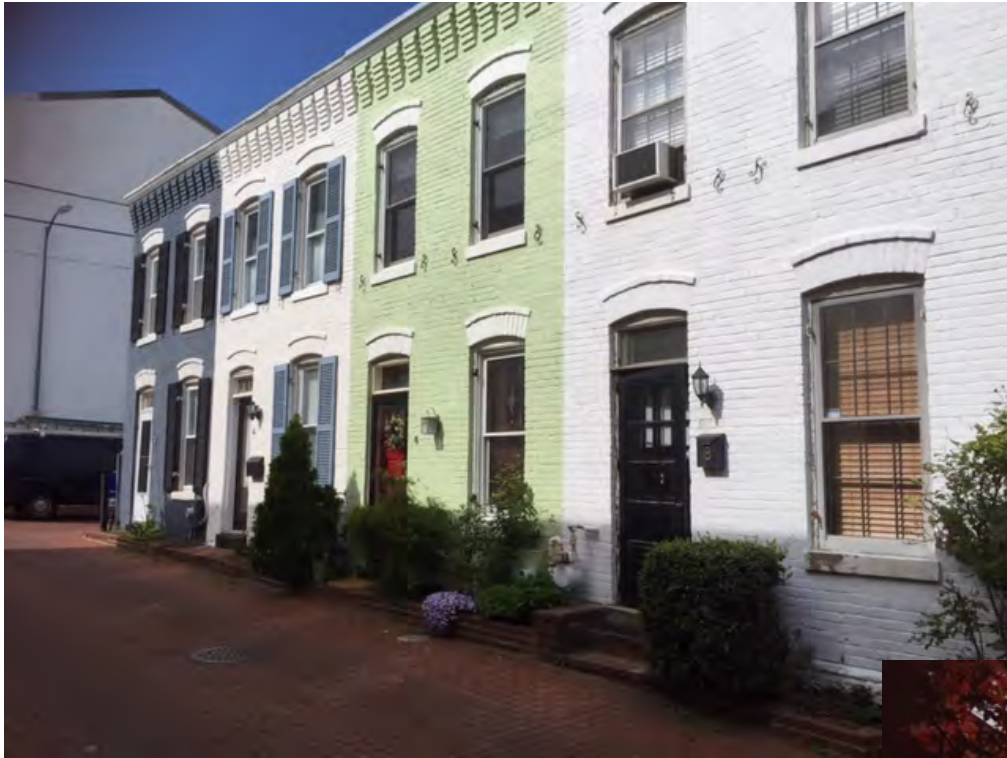
VIEW OF TERRACE COURT
