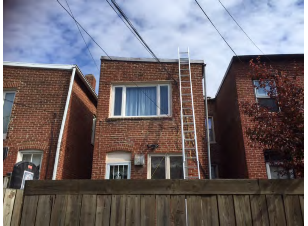
REAR OF 215 A STREET NE
