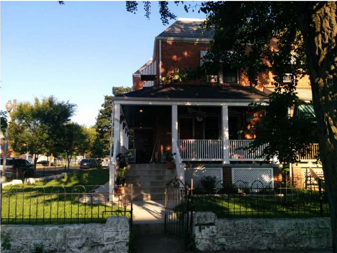
Street frontage of 1329 Holbrook St. NE, View from Holbrook St.
