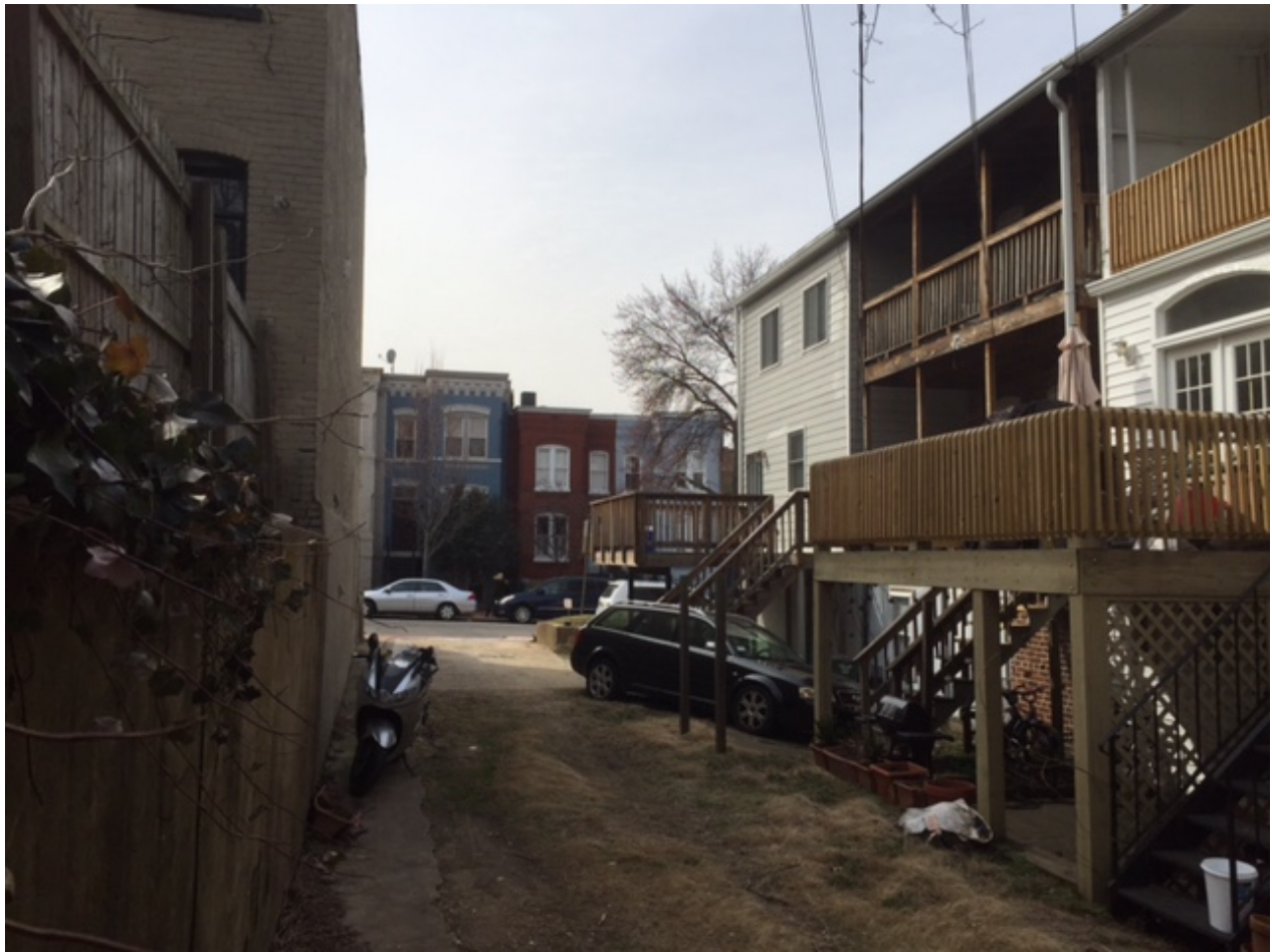
REAR VIEW, LOOKING WEST
