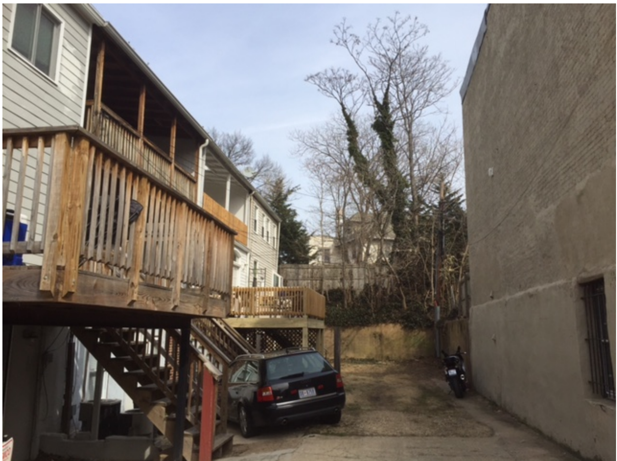
REAR VIEW, LOOKING EAST
