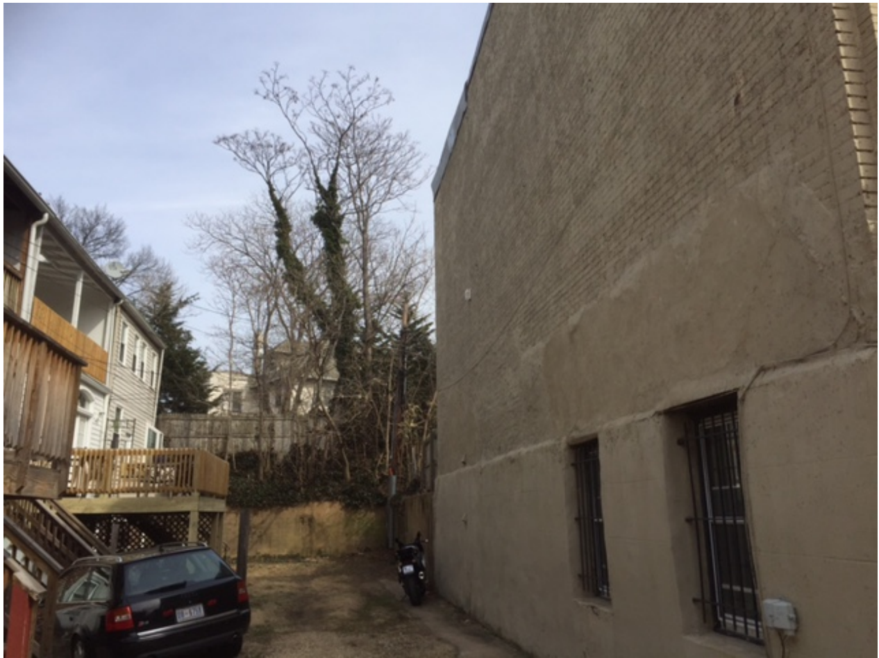
NORTH WALL OF PROERTY ON 10 TH STREET NE
