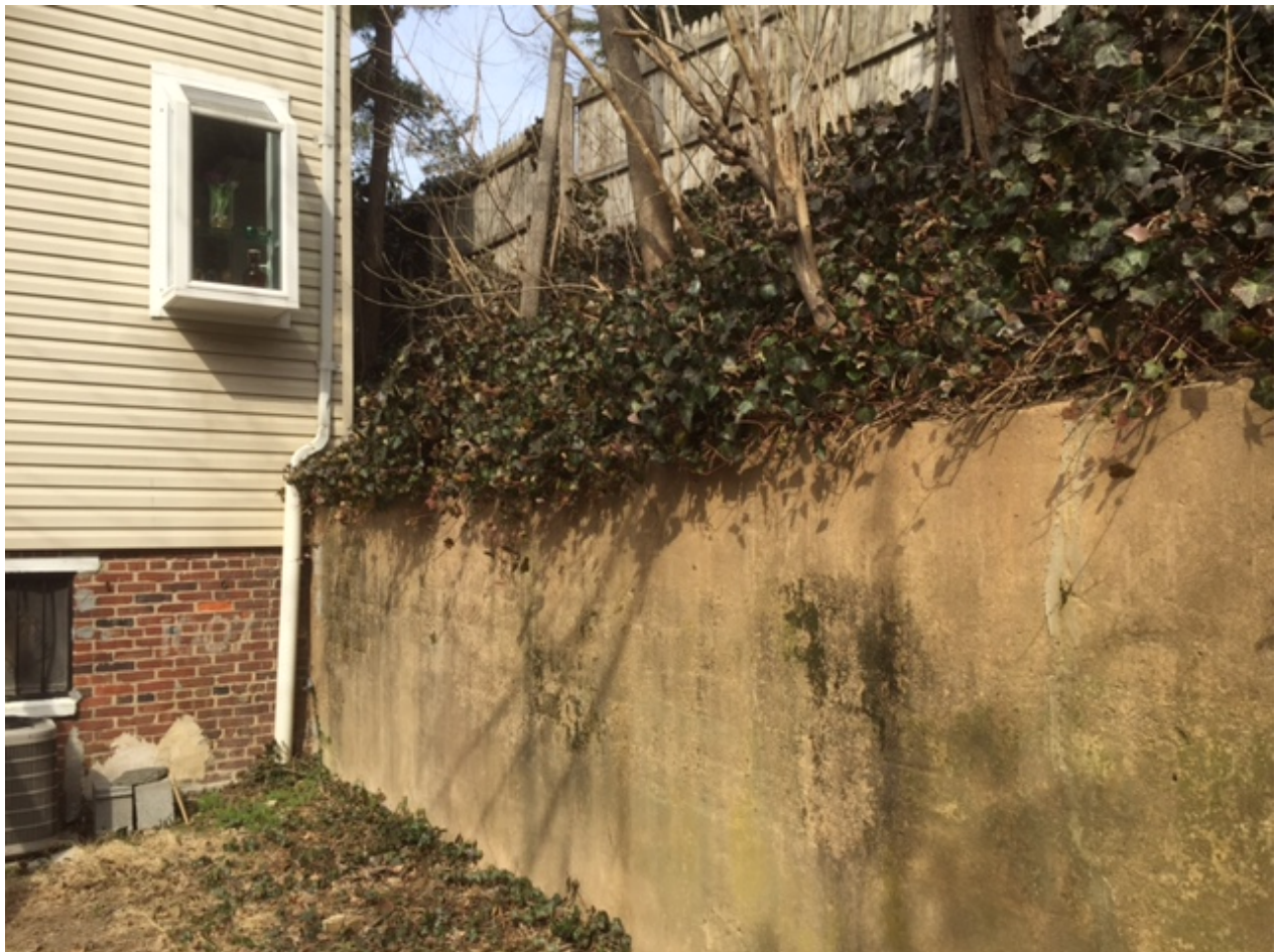
EXISTING WALL ALONG EAST PROPERTY LINE OF 1007 F STREET NE
